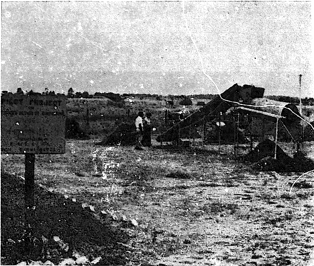
19. Pilot project for manual composting at Bangalore. Input is about three tonnes/day and the processing time up to 20 days.
