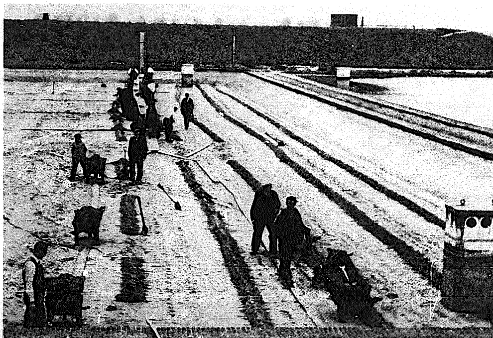
Municipal waterworks, Amsterdam
