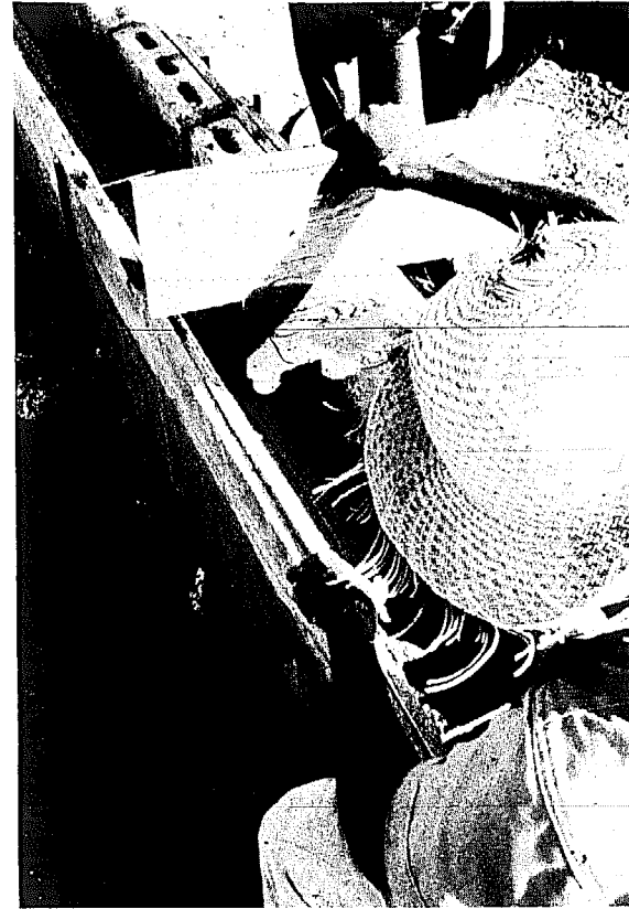
Fig 4: Specially contoured wood and metal backed mould used in forming the fine finish on the gutters
