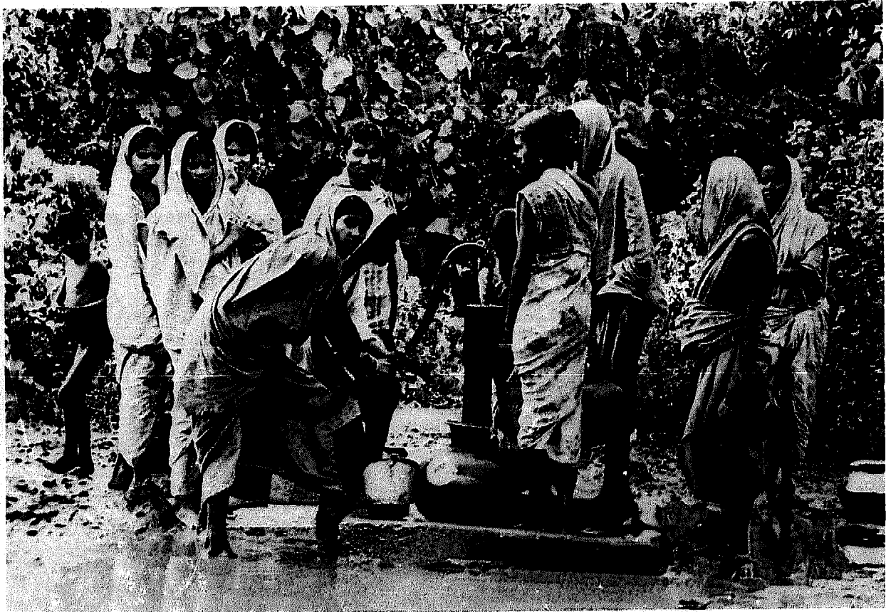
FIGURE 4-3 HAND PUMP WITH INADEQUATE DRAINAGE
