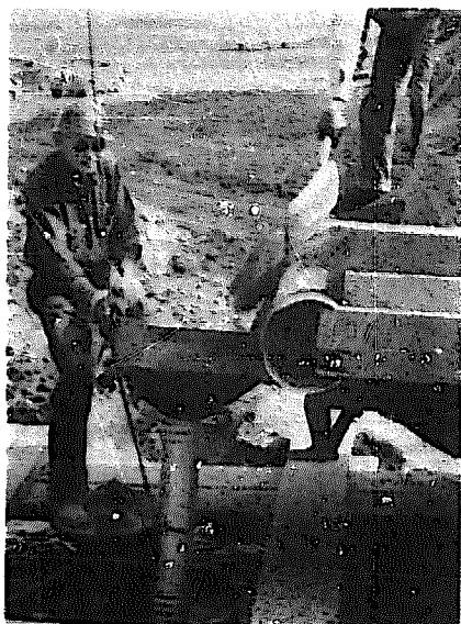
Fig. 5.37 PLACING GRAVEL-PACK MATERIAL THROUGH PIPE USED AS TREMIE.
