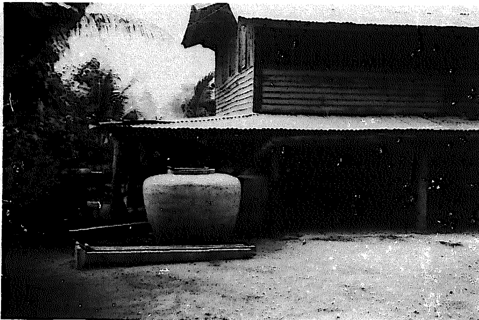
Figure 5.1. Simple roof catchment and storage (Thailand)
