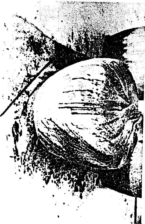
2.6 Spray some water on the mould before plastering to make it damp.
