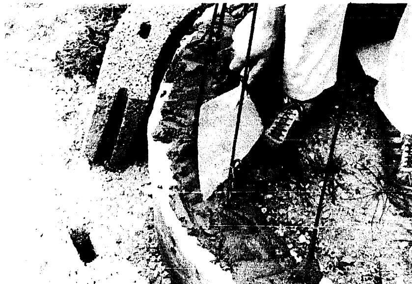
Photo 70 d) Check cutting ring starter bars and crank them into place if necessary. Attach vertical re-rod, trowel mortar onto ring and fit blocks over re-rod. (Caisson built above ground for demonstration purpose).
