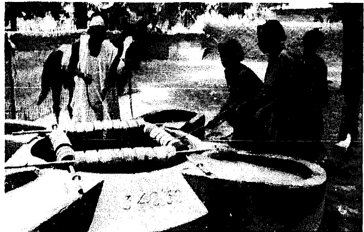
Photo 27 Nigerian Wellhead with Wooden Rollers – Northern Nigeria.
