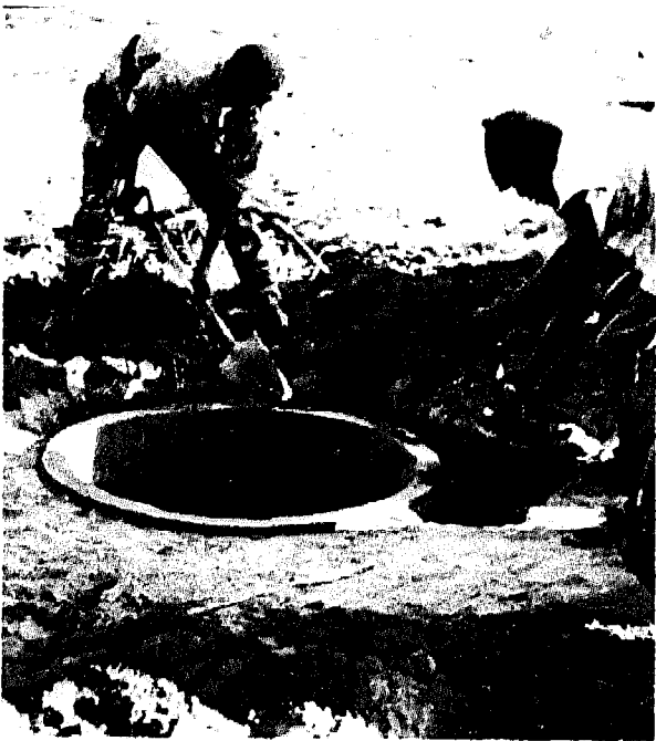
Photo 42 Digging up the casting.
