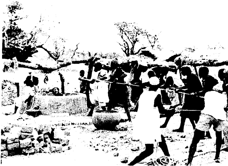
Photo 35 Lowering man down the well. The improvised headframe is made from local timber. – Upper Volta.
