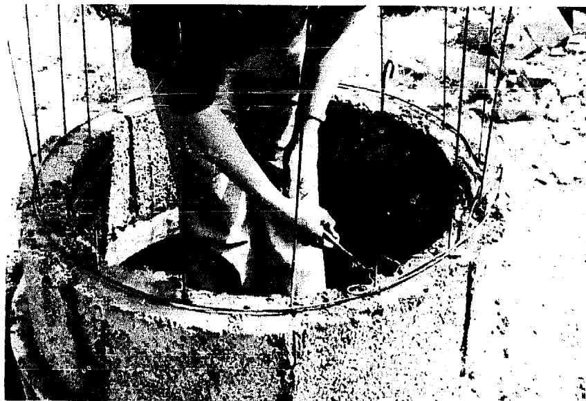
Photo 72 f) On every course of blocks a horizontal re-rod is tied, laid on a bed of mortar and the next row of blocks laid.
