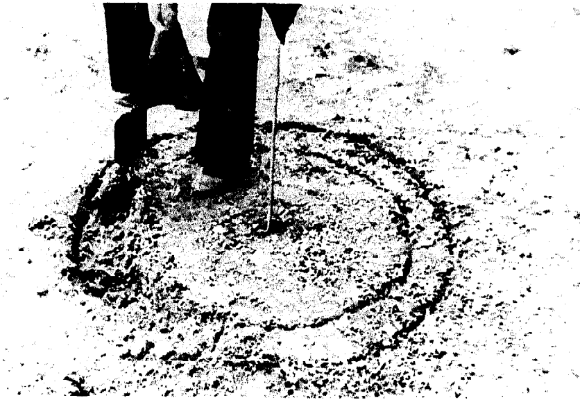
Photo 60 Making the Cutting Ring Without a Mould – a) Mark out ring on ground and dig roughly to size.
