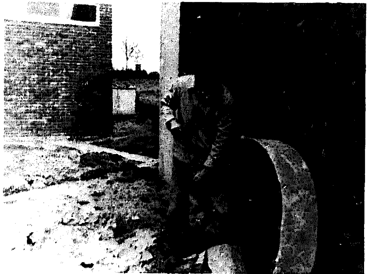
Photo 66 g) Leave ring one week to cure then dig out and clean.
