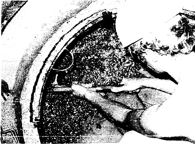
Photo 57 Preparing the Cutting Ring Ready for the Pre-cast Blocks — c) When cutting ring has cured, remove mould sections by excavating below ring.
