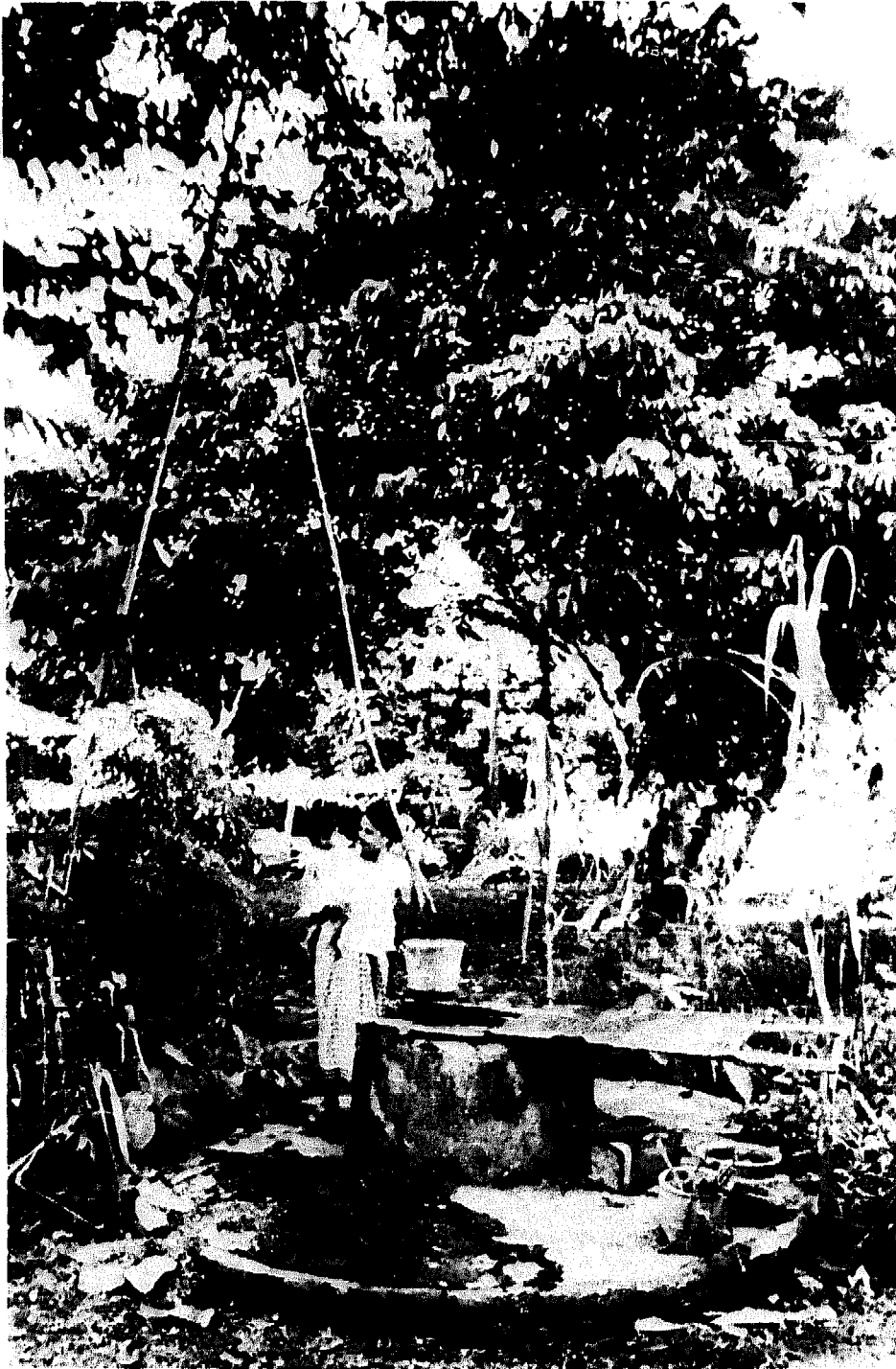
Photo 5 Protected well with sliding cover and Shaduf water lifting device.
