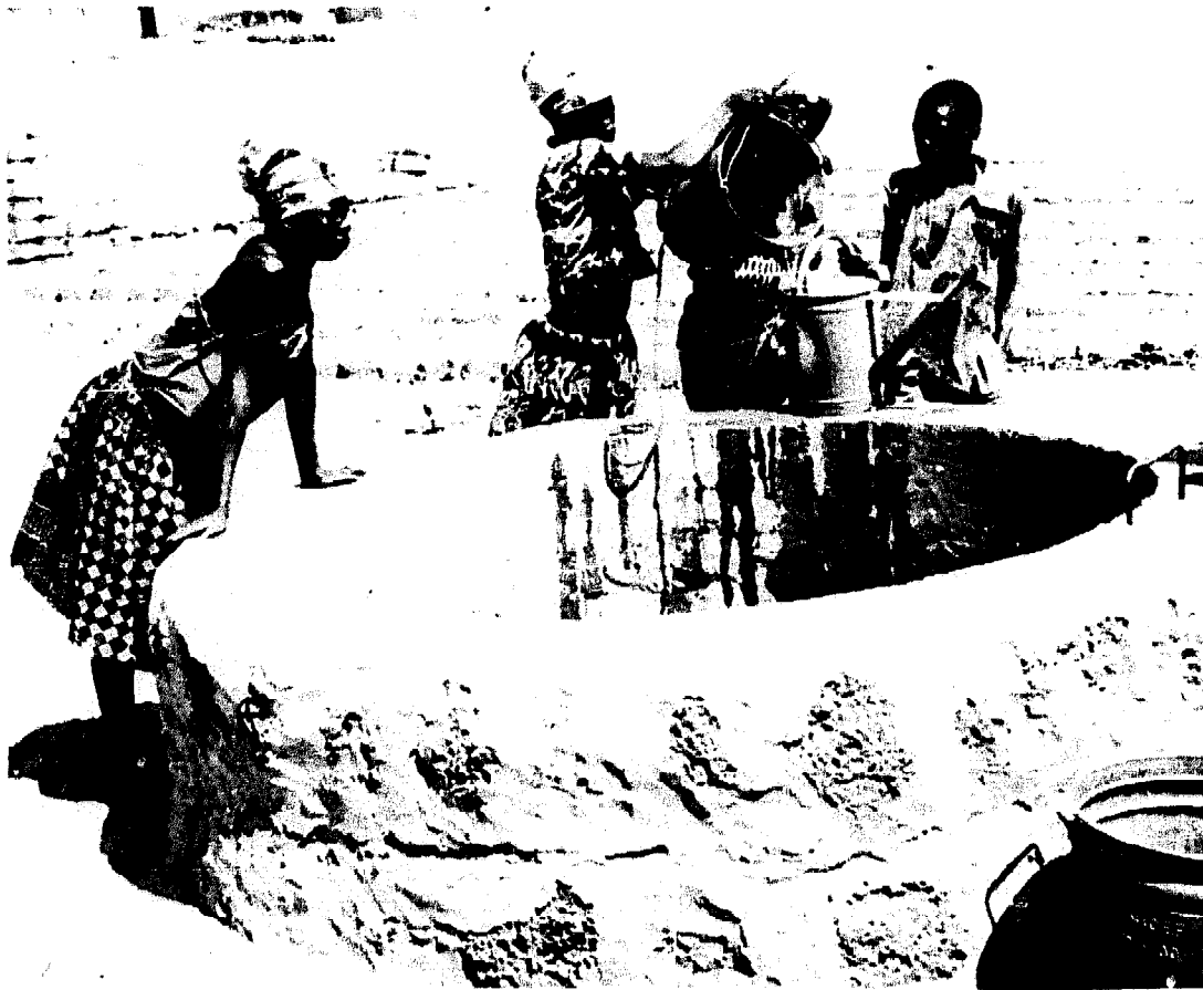
Photo 45 Masonry Lined Well – Upper Volta.
