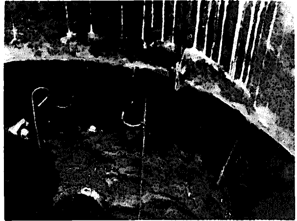
Photo 17 Placing of re-rod begins. Note the hooks and overlap.
