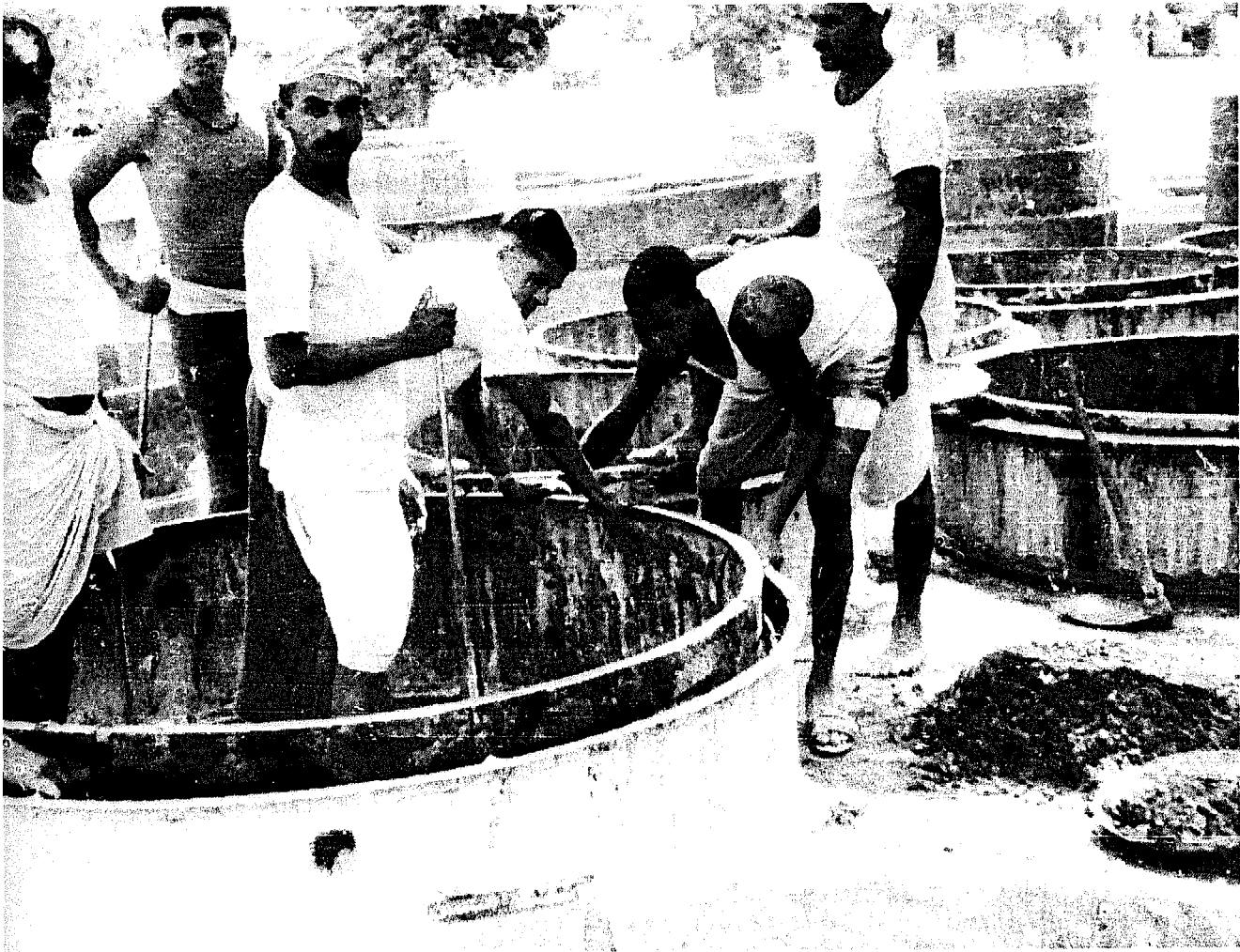
Photo 24 Caisson ring mould 0.5 metre deep – c) Making concrete rings. – India.
