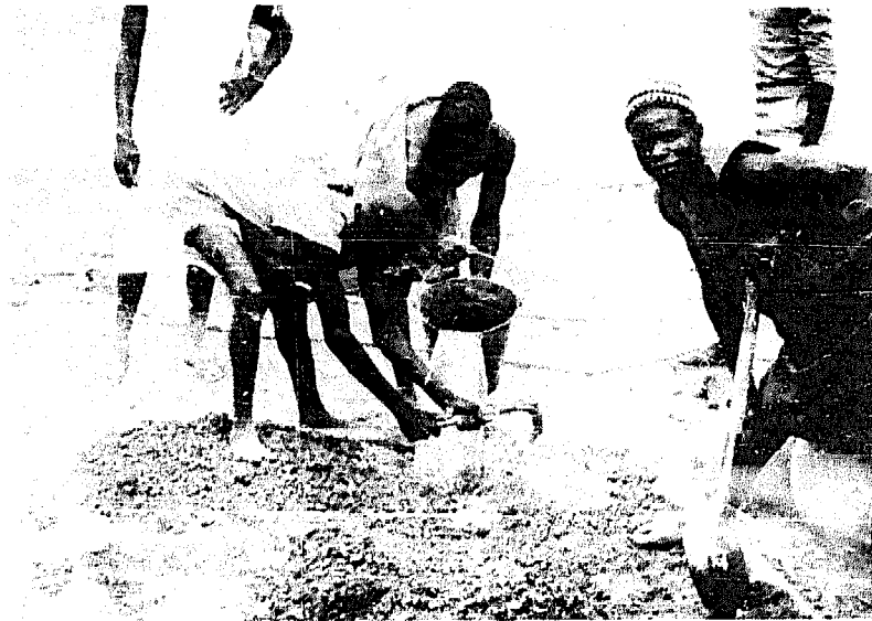
Photo 14 Mixing the Concrete by Hand on the Mixing Tray — Low walls prevent accidental loss of cement slurry. In the photograph a hoe is being used; square shovels make the work easier. — Upper Volta.
