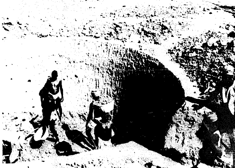
Photo 4 d) Excavating 10 metre diameter well and removing spoil up a ramp cut into the side of the well. Well excavated into slow flowing aquifer. — India.
