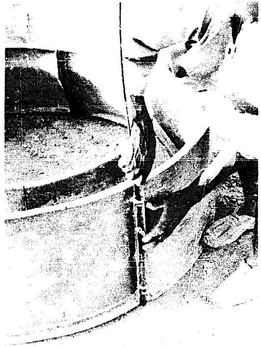
Photo 52 Building Up The Cutting Ring Mould – d) Removeable wedges to loosen sections for removal. – Upper Volta.
