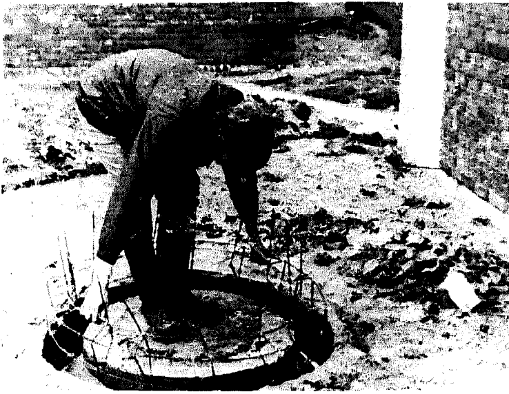
Photo 64 e) Wedge frame to shape using pebbles, then tie frame securely. (right)
