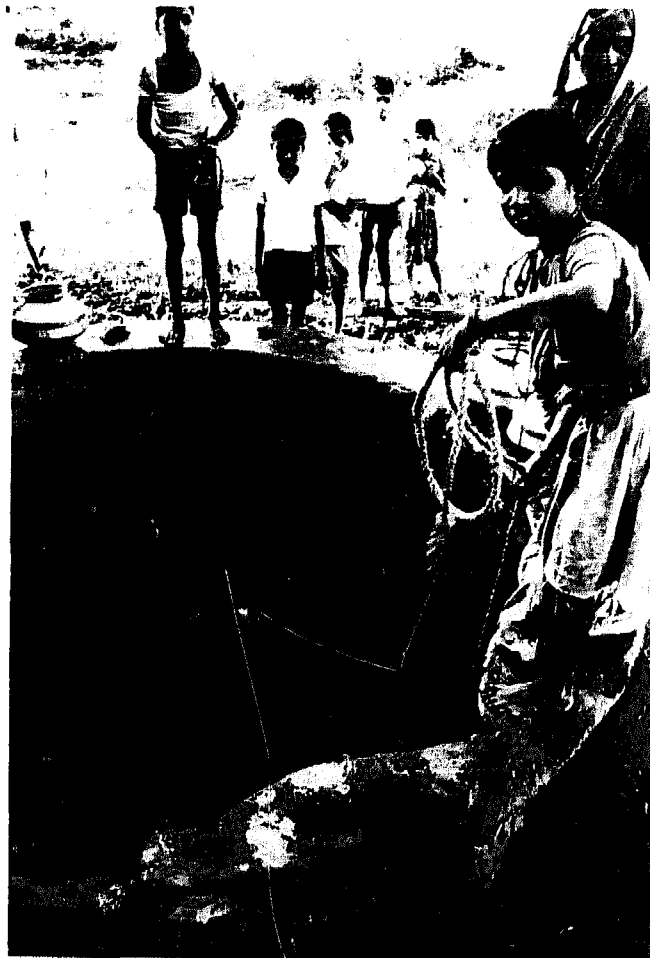
Photo 7 b) 3 metre diameter hand dug well brick lined with a low headwall. Sullage water is tipped by the wellhead -- the users carry contamination onto the wall on their feet and this drains down into the well. This well can be improved by constructing a drainage apron and making the headwall too narrow to stand on. -- India.
