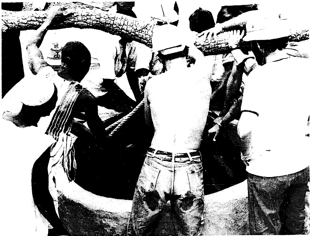
Photo 54 f) Lower assembled sections into well. – Upper Volta.
