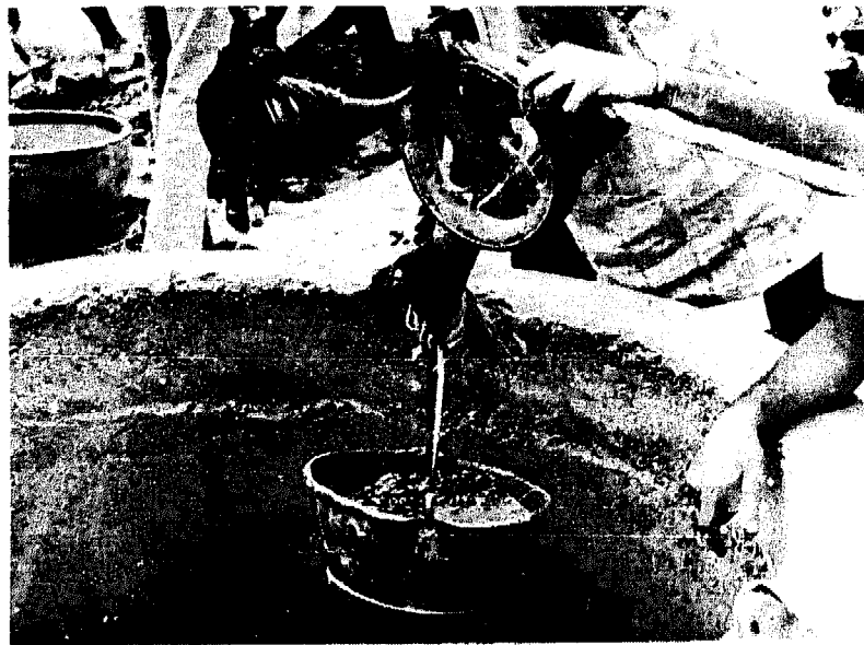
Photo 15 Lowering the Concrete into the Well in the Special Bucket — Upper Volta.
