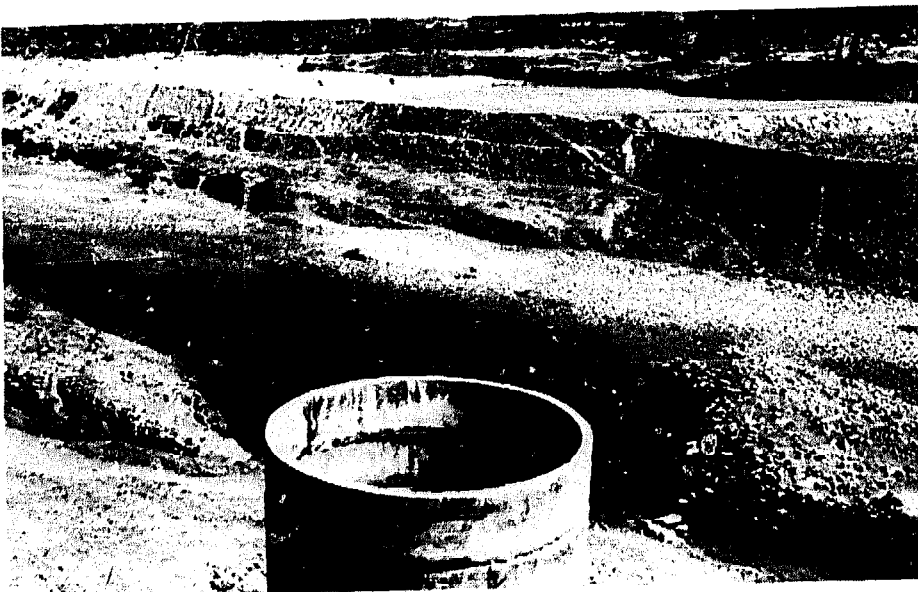
Photo 48 c) Caisson sinking a shallow well on the bank of a river will give a clean and plentiful supply of water.
