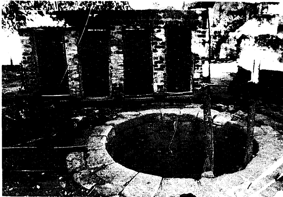
Photo 6 Wellhead Contamination -- a) New latrines built alongside a well which will be abandoned. Even if the well is filled in, the aquifer is still liable to be contaminated. -- India.
