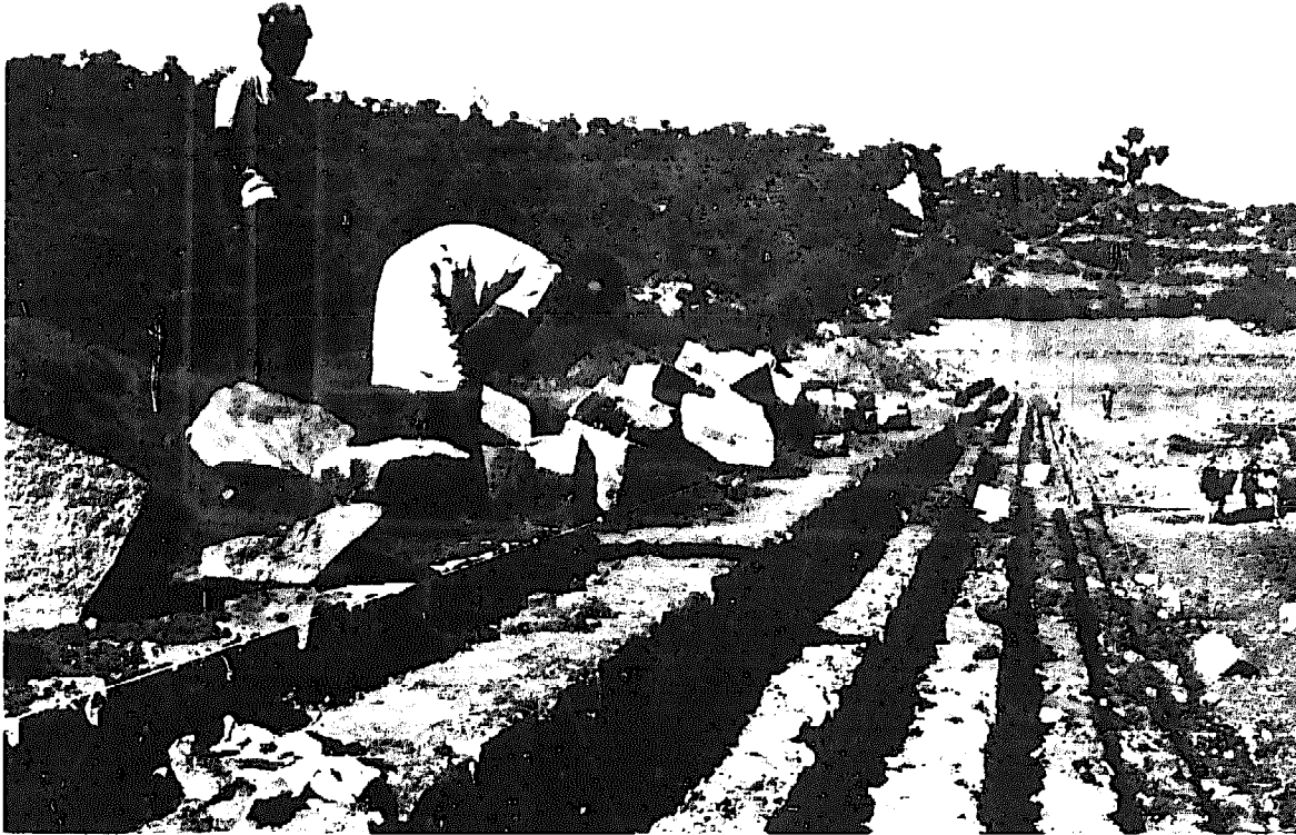
Fig. 11. Stone-faced earth dam for water conservation under construction at Otterthotti, in the Karnataka state of India. (photo: Father Godest).
