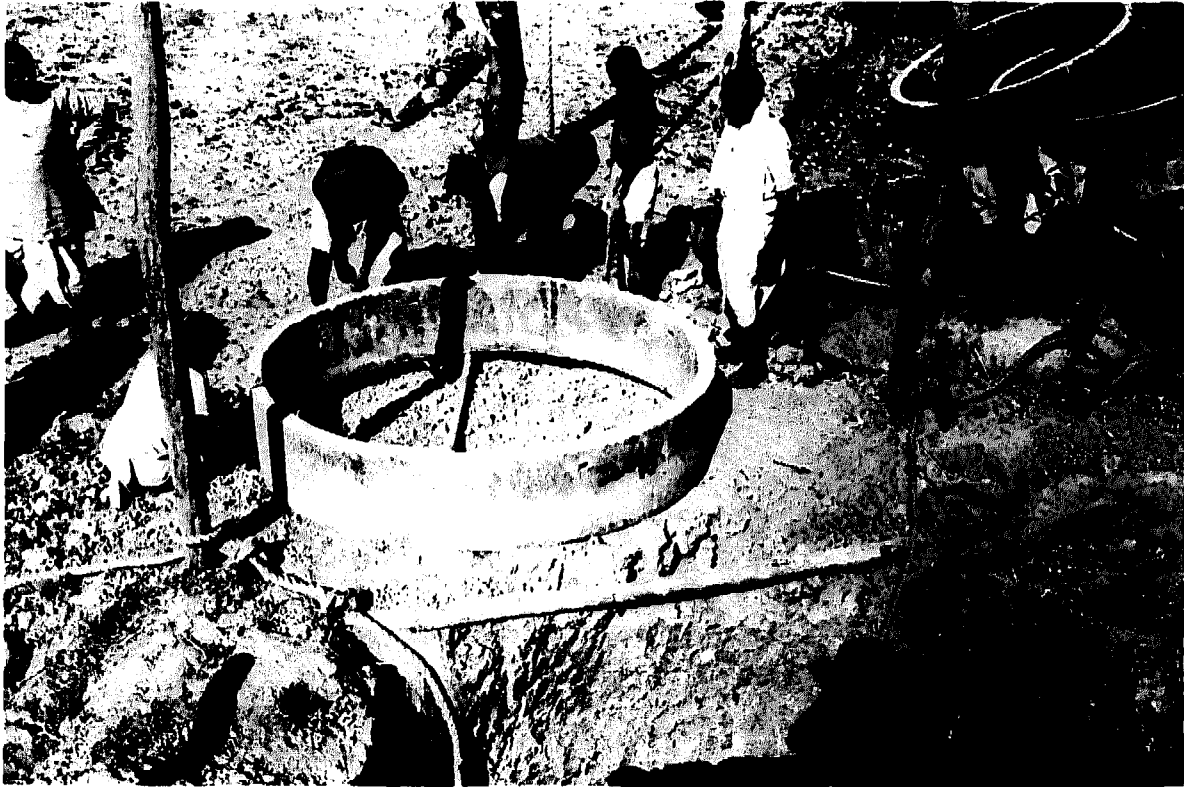
Fig. 5. Pre-cast concrete rings for lining a well in Bihar, India. (photo: Jim Cranmer/Oxfam.)
