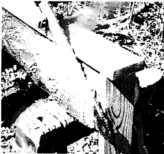
Keep the logs in sets of four — 2 cross and 2 filler for each course.
