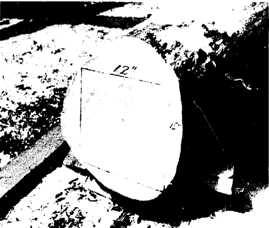
Transfer this square using these measurements to the other end of log. Use the level to "true".
