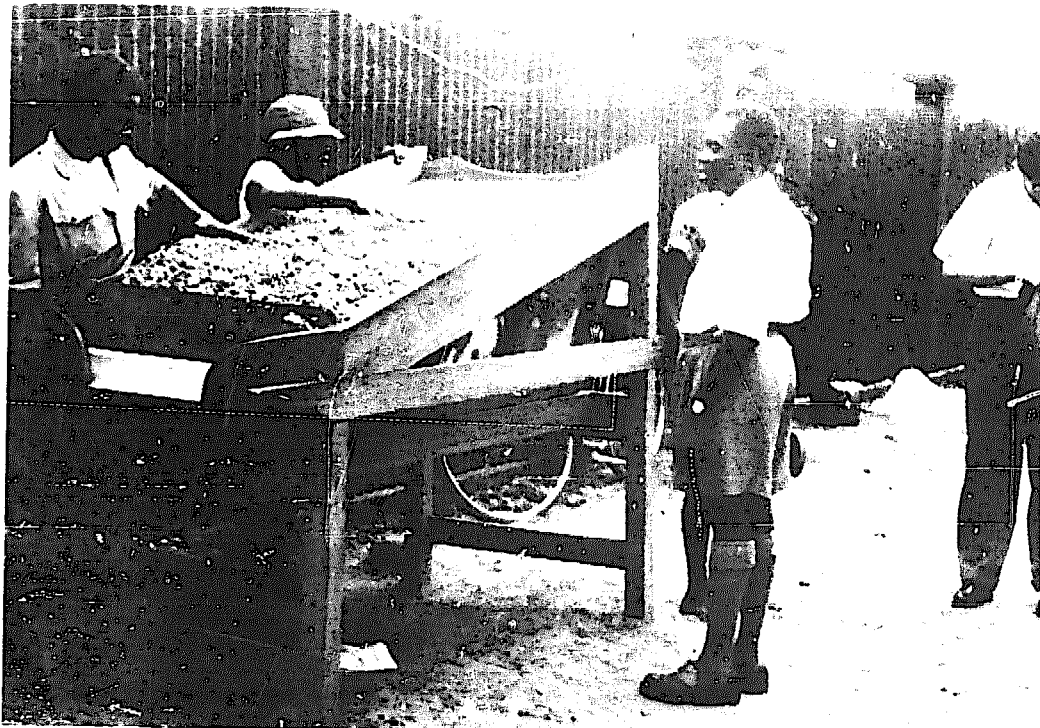
FIGURE 18. Simple types of sampling methods. Above, snaking, below, sieving.
