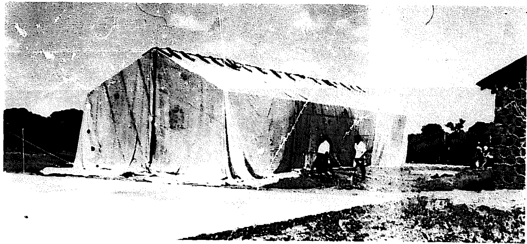
FIGURE 58. Enclosing an entire warehouse in gasproof sheets for purposes of fumigation.
