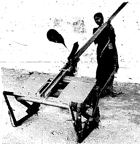
Fit the beam on the channel assembly ...
