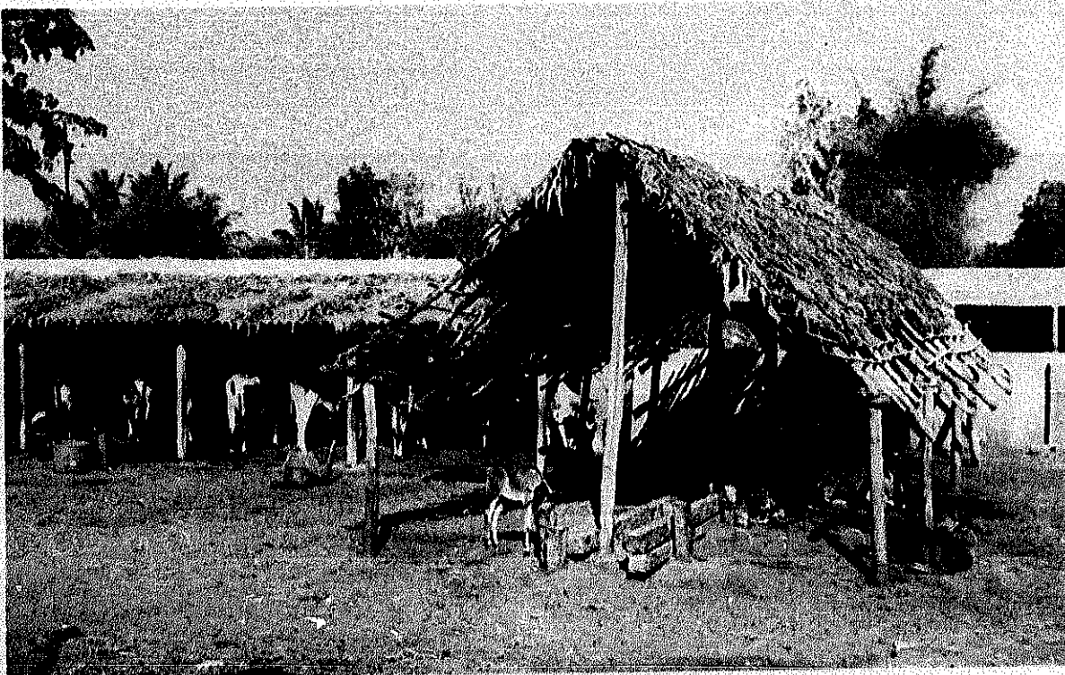
Fig. B/I/6: Shade-providing roofs made of local materials usually fulfil the requirements for draught-cattle housing and are also cheap to erect. (Photo: Reh)
