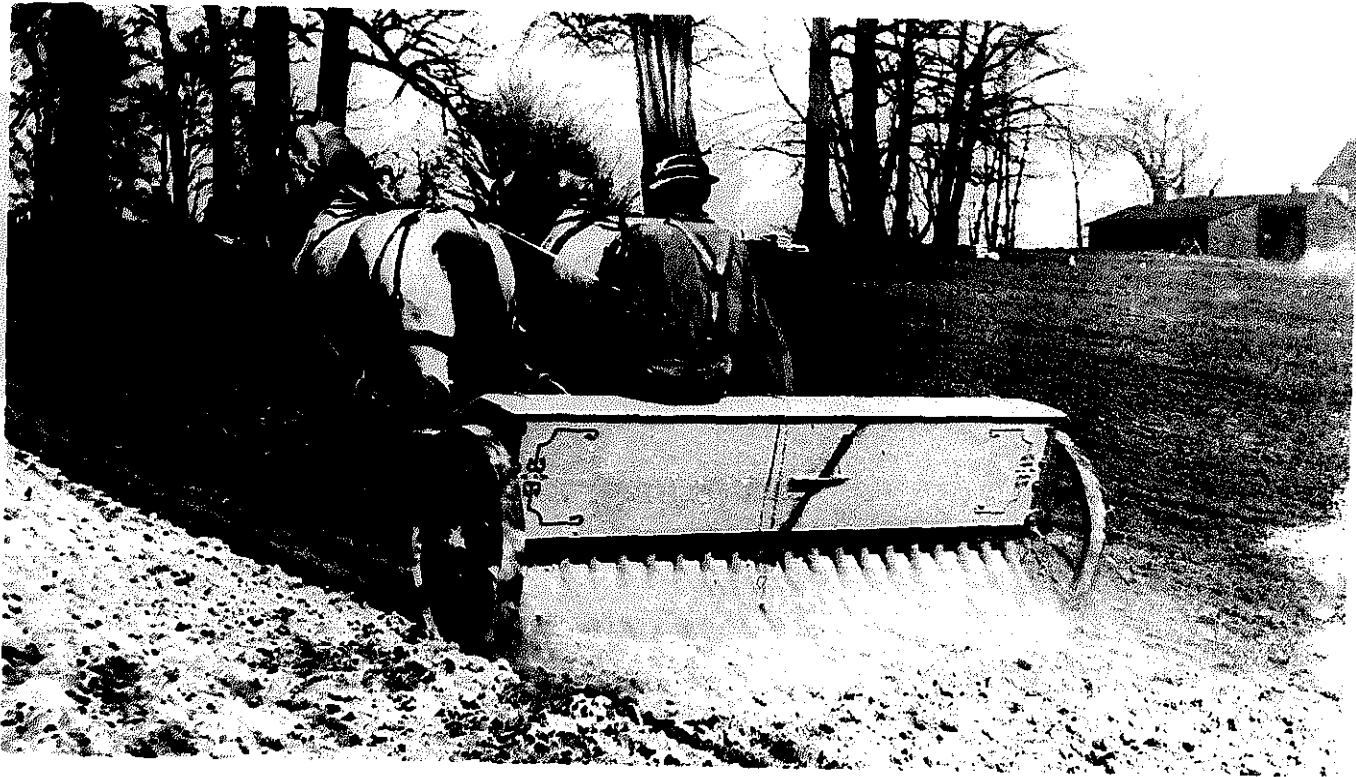
Above: During the 1860s, implement manufacturers began adding the force-feed mechanism to the box seeder or sower. The force-feed mechanism deposited a uniform amount of seed or fertilizer through the tubes. Here, a force-feed sower evenly spreads fertilizer across the field. (Smithsonian Institution.)
