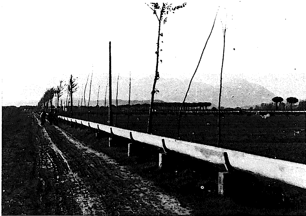
FIGURE 23. Precast concrete flumes mounted on pedestals carrying water to irrigated fields.
