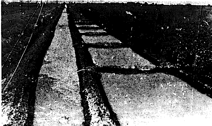
FIGURE 77. An auxiliary ponding area used with furrow irrigation. A siphon delivers the water into the ponded area, and spiles release the water from the ponded area into the furrows.
