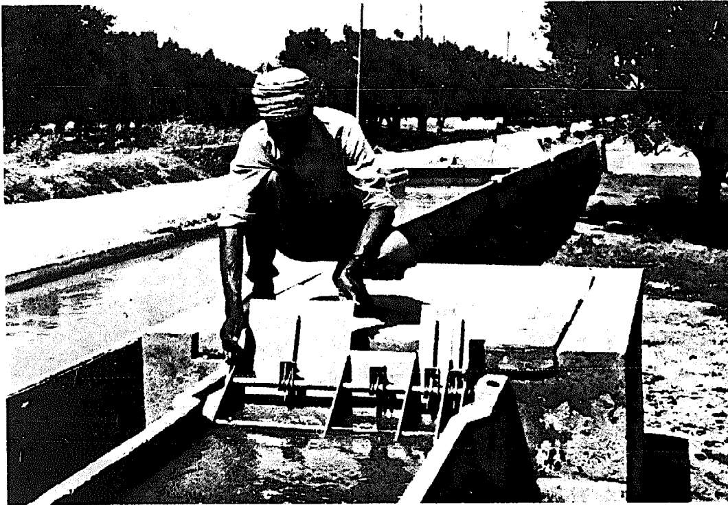
FIGURE 1. Distributor, with Neyrpic automatic gate downstream in the main canal to regulate water depth.
