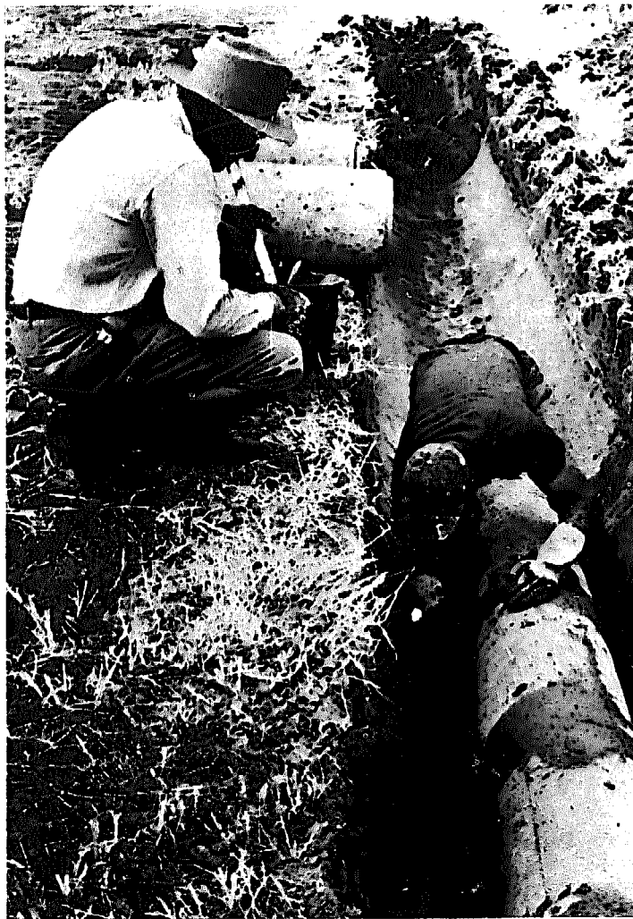
FIGURE 34. Workman installing precast concrete pipe in trench.
