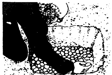
2 Put a layer of stones in the bottom of the hole to help with drainage.
