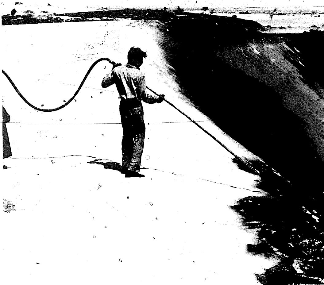
FIGURE 53 Stabilizing dunes with a heavy oil mulch in the Rajasthan Desert, India. This process was first applied in Libya to 160 ha of bleak, barren stretches of the Sahara Desert (see also FIGURE 55). The dunes contained moisture 0.5 m below the surface. After treatment they were planted with 60,000 eucalyptus trees; 90 percent survived the planting and continued to grow. One m high when planted, they grew to over 2 m during the first year. Unstabilized sand would either bury the young plants or blow away, exposing their roots. (Exxon)
