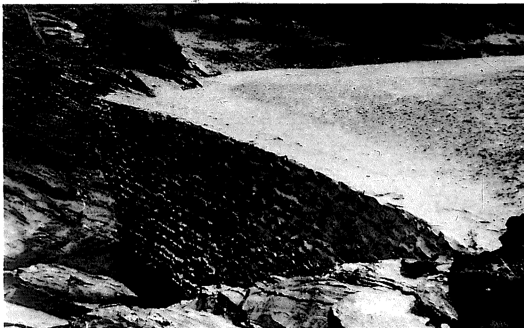
FIGURE 45 Sand dam in South-West Africa built of rock and mortar. (O. Wipplinger)
