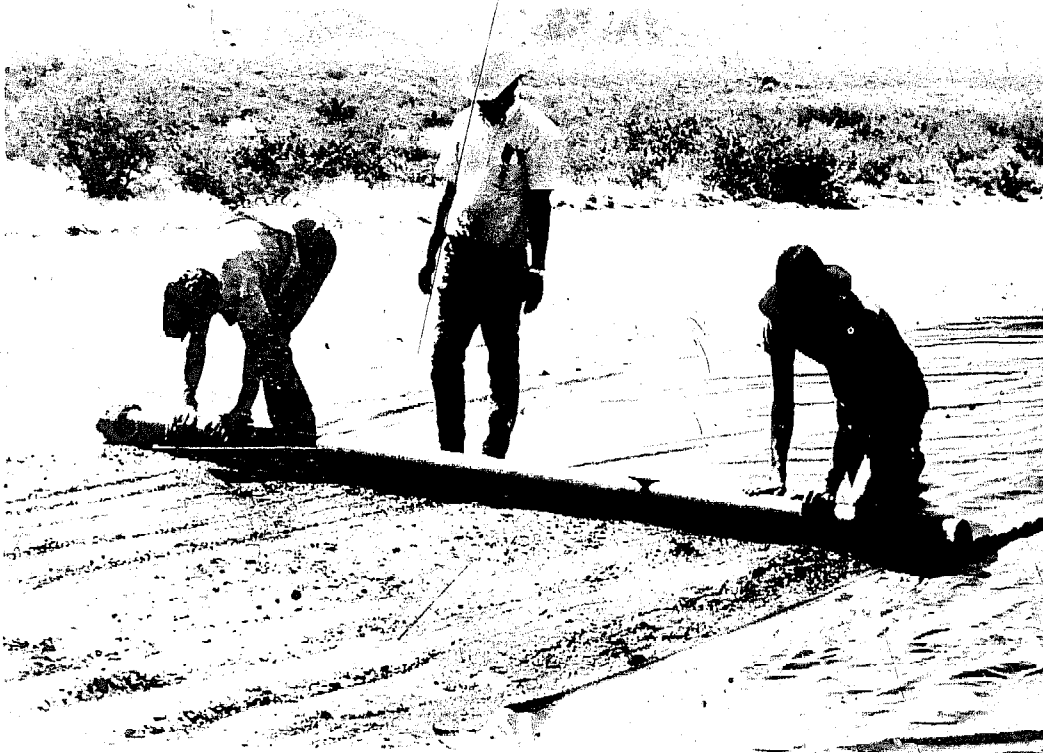
FIGURE 9 Laying polyethylene sheet for a rainwater catchment in the Sonoran Desert, Arizona, USA. Sheet was later covered with gravel for protection against damage and sunlight. (C.B. Cluff)
