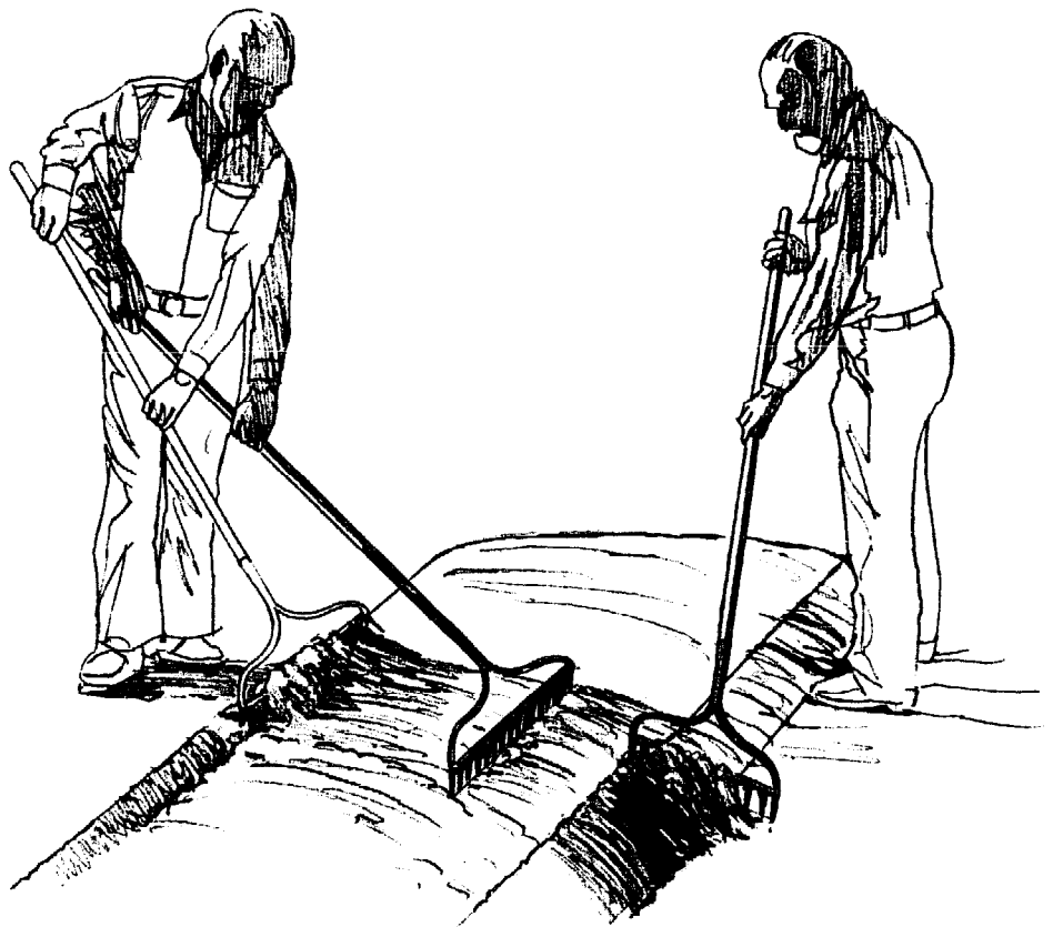
(Left) raking soil outward from inside for lip. (Right) raking soil up from side for lip.
