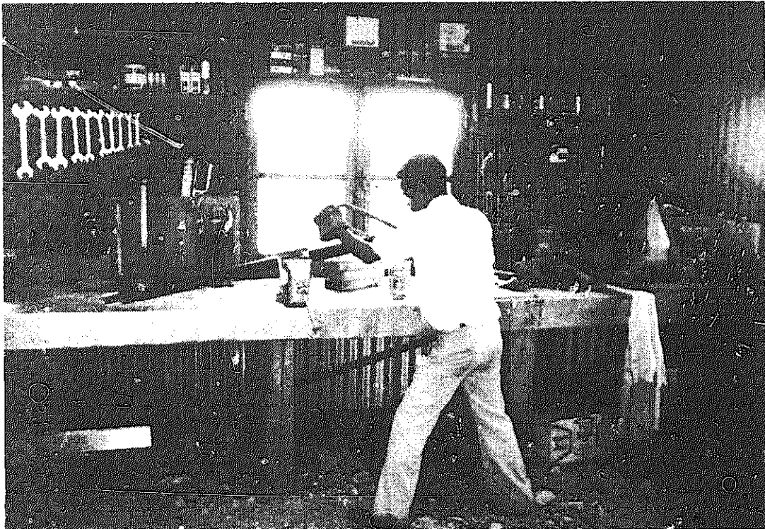
Cutting angle iron in the Garage workshop. (Photo: ITDG).
