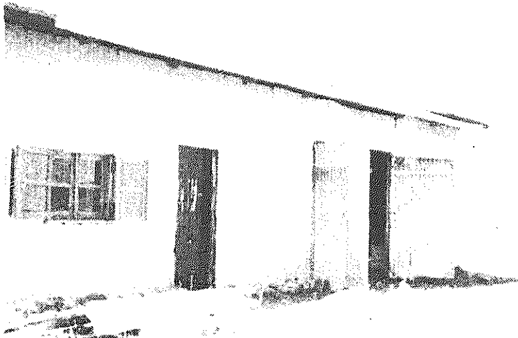
Garage Water Development Project workshop in Ethiopia. Originally this workshop had only two window openings and one narrow door. It was improved to include seven glazed windows, with shutters, alternating skylights on both sides of the roof slopes, and a pair of double doors. (Photo: S. Bonnist).
