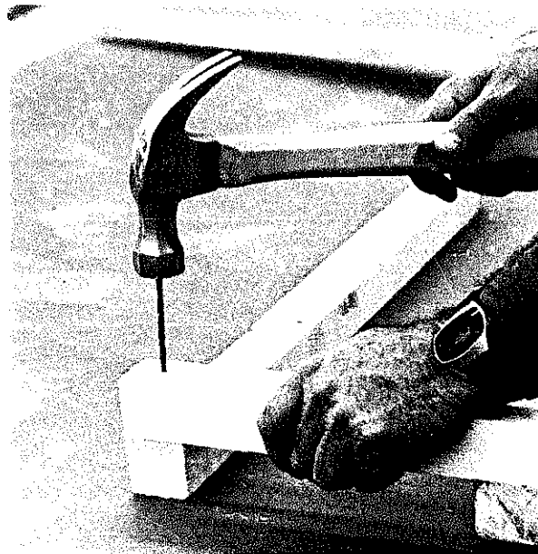
Fig. 11-25 Starting a nail.
