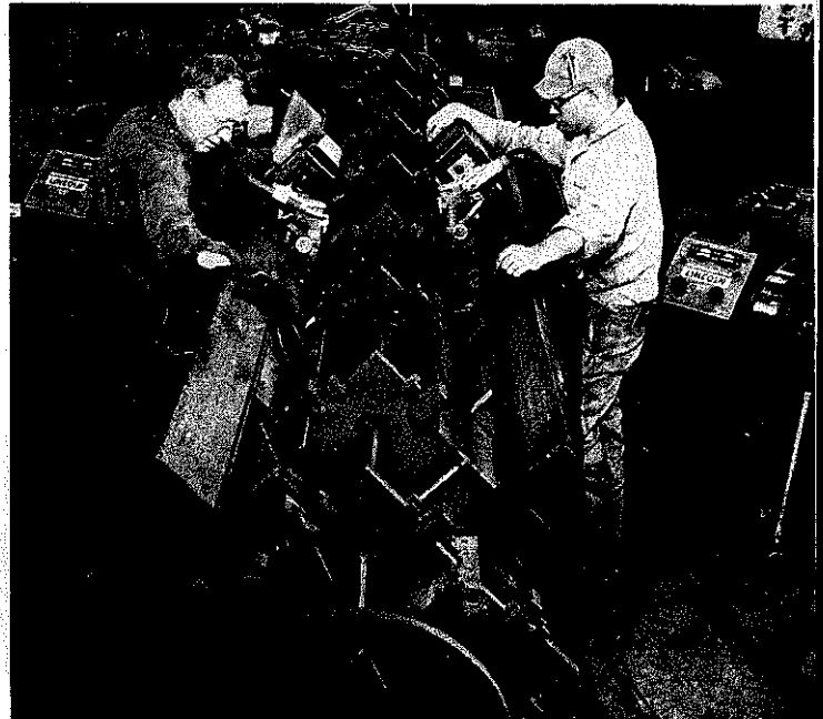
Operators work on a tandem fixture to make 3/8 inch fillet welds on low-alloy, high strength "T" sections for a water reservoir structure. They are using a trackless tractor that develops full mechanized welding performance while featuring extreme portability and simplicity.
