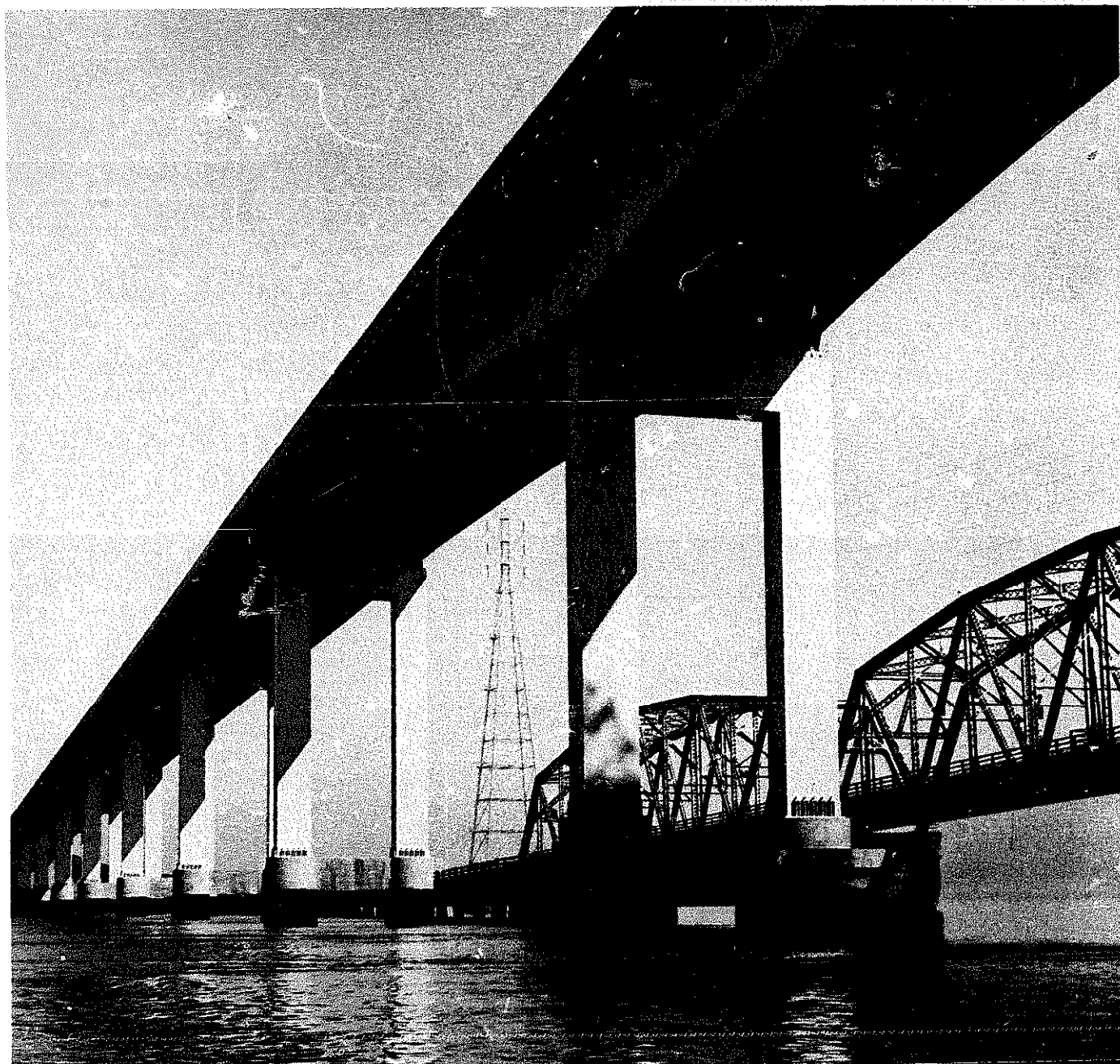
San Mateo-Hayward (California) bridge. Note the old and new structures. See page 13.2-3 for the fixture used to weld the columns.
