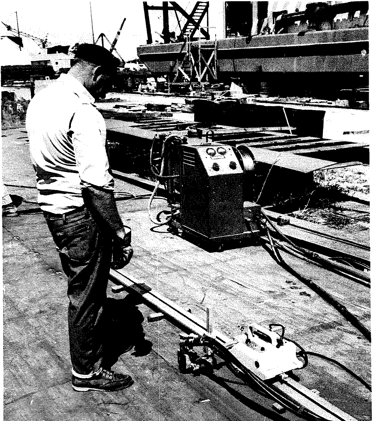
Splicing deck plate with mechanized submerged arc welding. Mechanized welding is an aid to minimize distortion.
