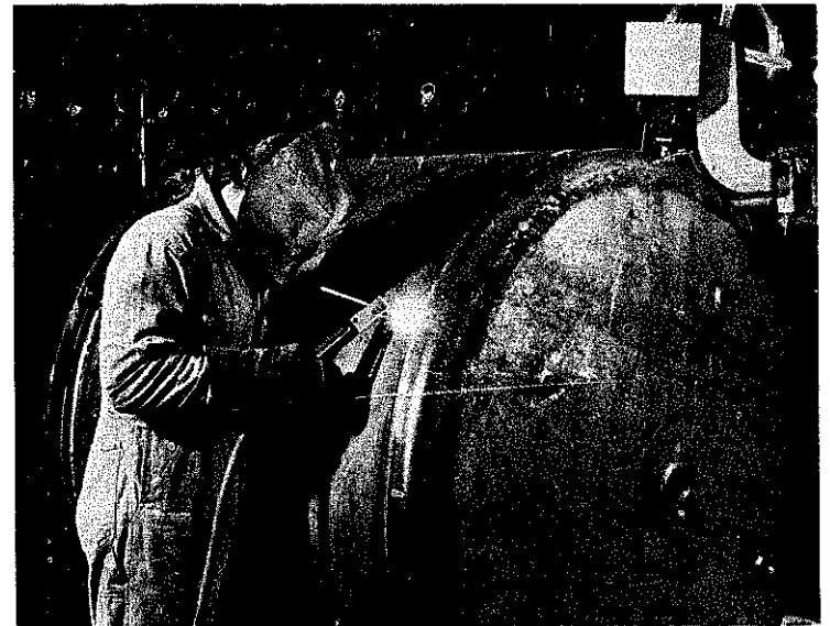
Fig. 13-31. Back-gouging of a seam welded from inside the tank as preparation for a weld to be made from the outside.
