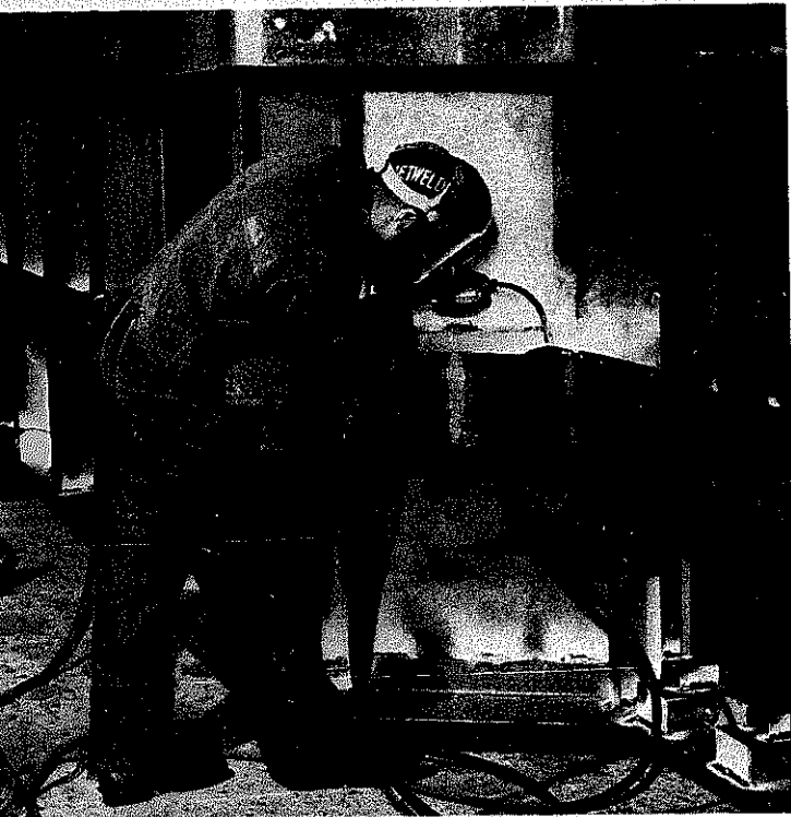
What the well dressed weldor should wear; a cap or hard hat depending on the job, safety glasses (not shown), head shield with the proper lens shade, leather jacket with long sleeves, leather gauntlet gloves, heavy trousers with no cuffs, and safety shoes.
