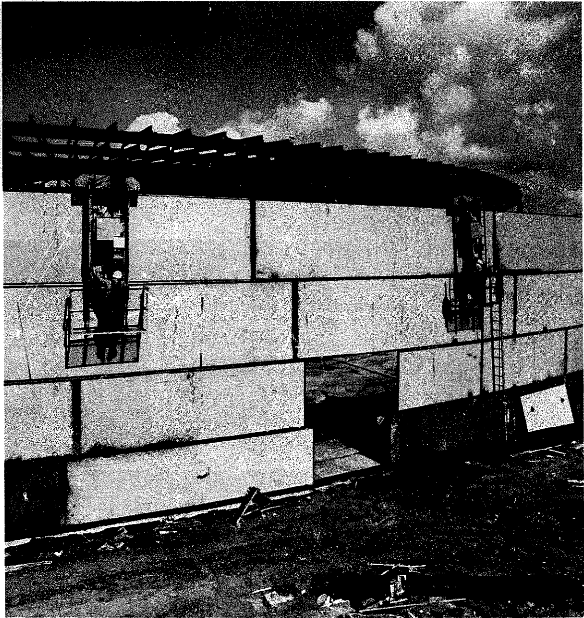
Welding horizontal seams on a storage tank with automatic open-arc process.
