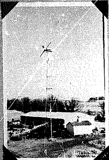
PHOTO 14. Air Electric 2000 Watt - 32 Volt - On Tower
