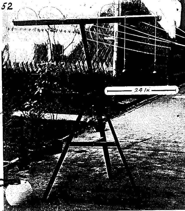
FIG. 260. TWISTING STAND FOR TWISTING COTTON THREAD.
