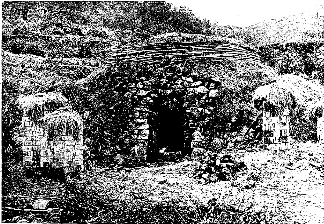
FIG. 392. KILN FOR BURNING BRICKS AND ROOFING TILES.
