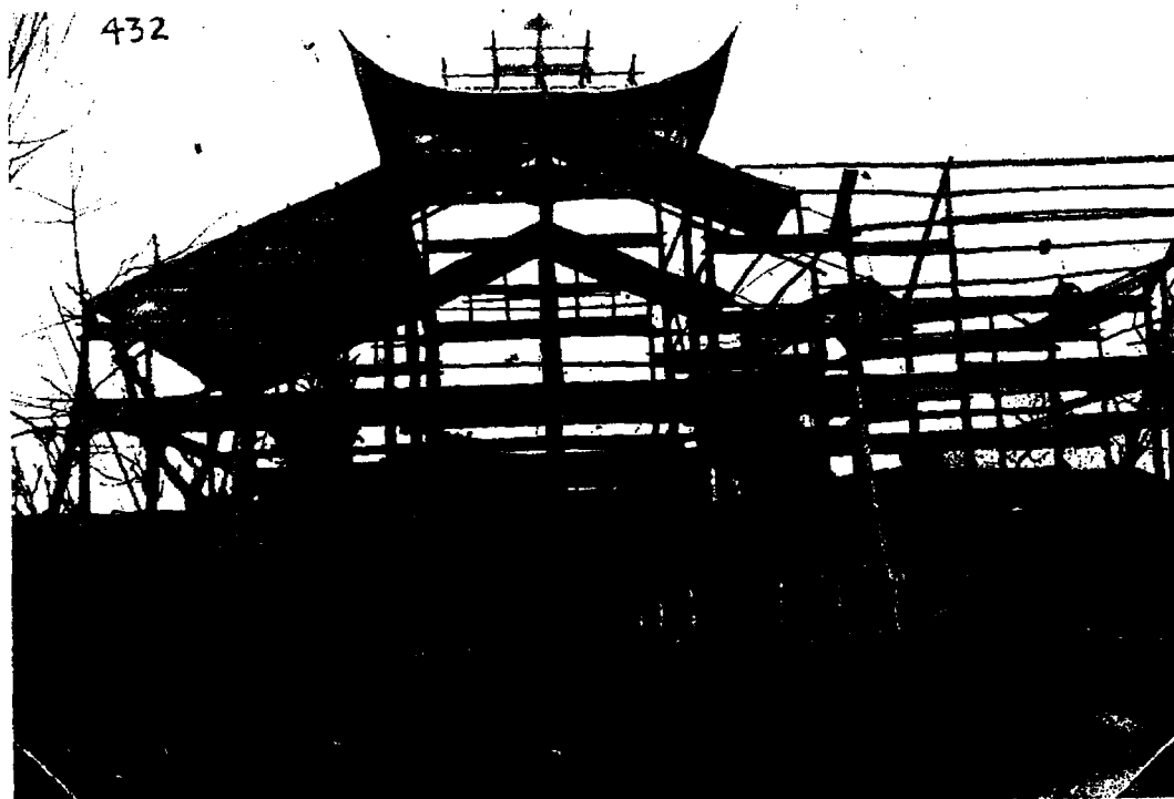
FIG. 416. WOODEN FRAMEWORK OF A TEMPLE IN COURSE OF CONSTRUCTION.
