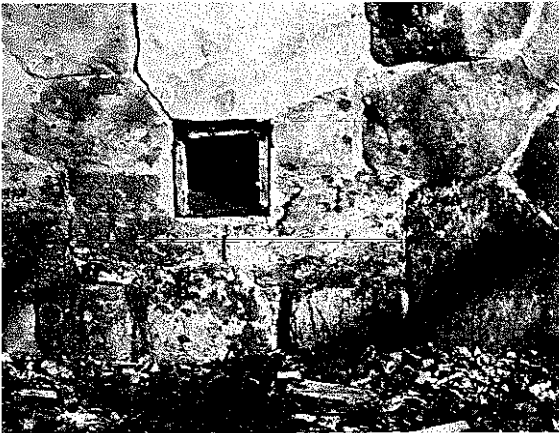
PLATE 320 Detail of the vent below the front door.
