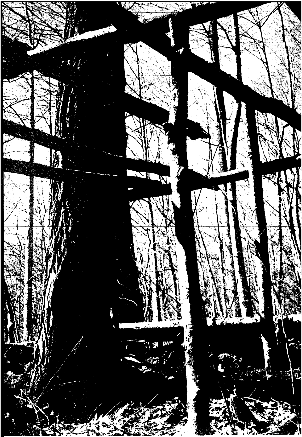
PLATE 260 This log framework was built in the woods to conceal a still. When finished, it was covered with branches.
