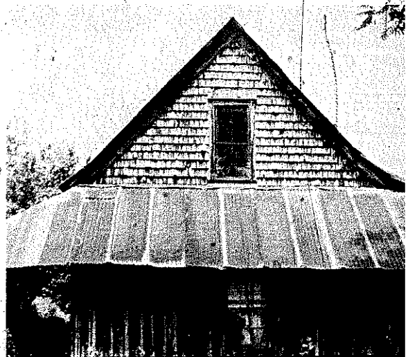
PLATE 117 A gable covered shingle fashion on a house near Franklin, North Carolina.
