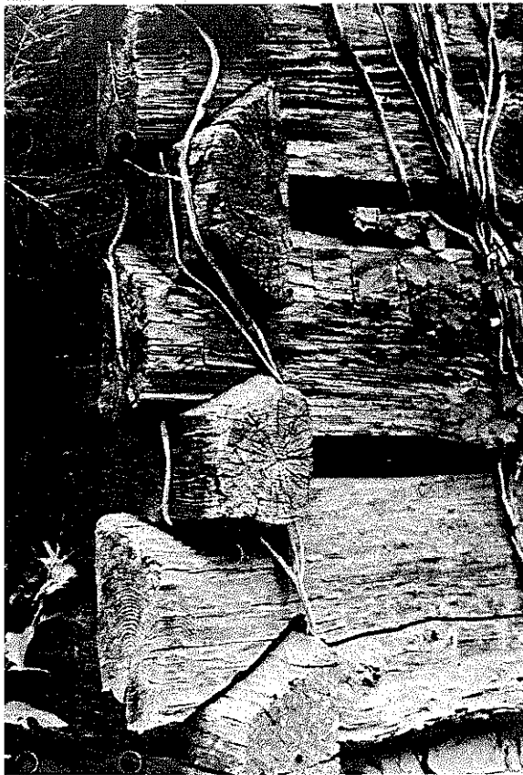
PLATE 85 Overhanging dovetail notches on the house built by Buck Carver's grandfather a hundred and fifty years ago. The house was torn down by its new owner in 1970.
