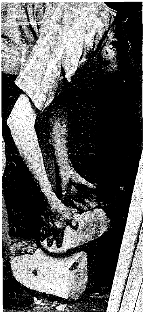
PLATE 66 Rest the next log, also hewed off on the sides, atop the first. Set it so its end is flush with the bottom log's side.
