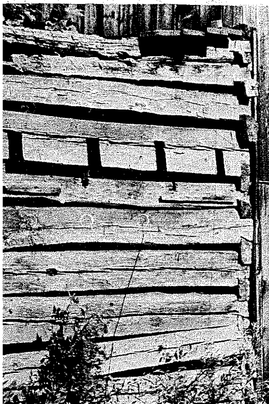
PLATE 95 In this building south of Franklin, North Carolina, the underside of the plate has been notched to accommodate each joist. Note the logs added above the plate to form a loft.
