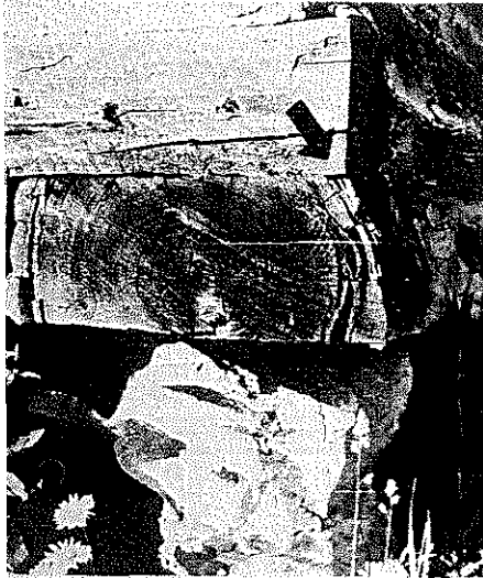
PLATE 60 The lap joint of this end log (arrows) fits snugly over the sill.
