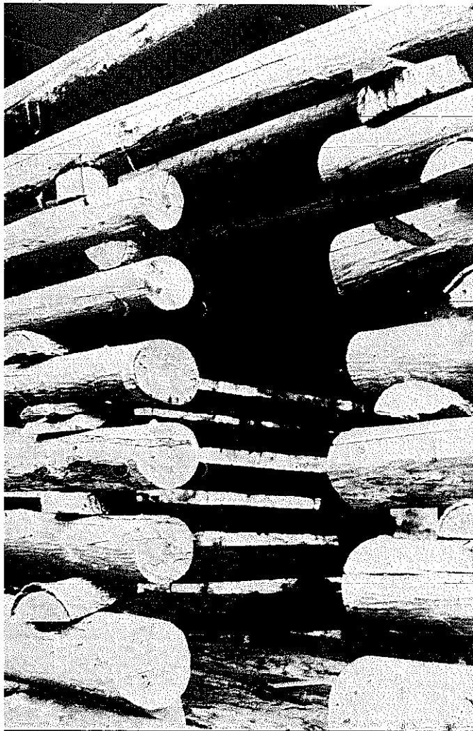
PLATE 132 The door opening on Thompson's cabin. Note the wedges between the logs to hold them up until the frames are added.
