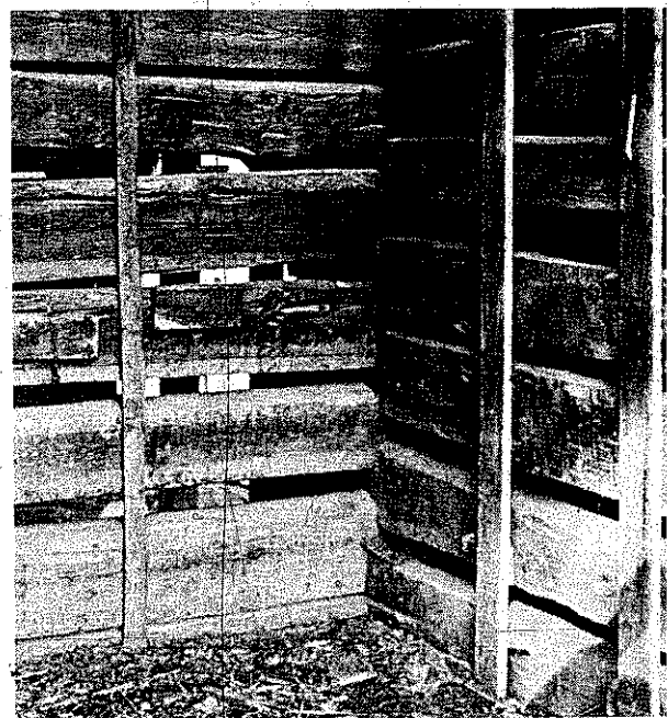
PLATE 89 The ends of this inside wall (running from left to center) have been notched to fit similar notches cut in the outside wall (running from center right).
