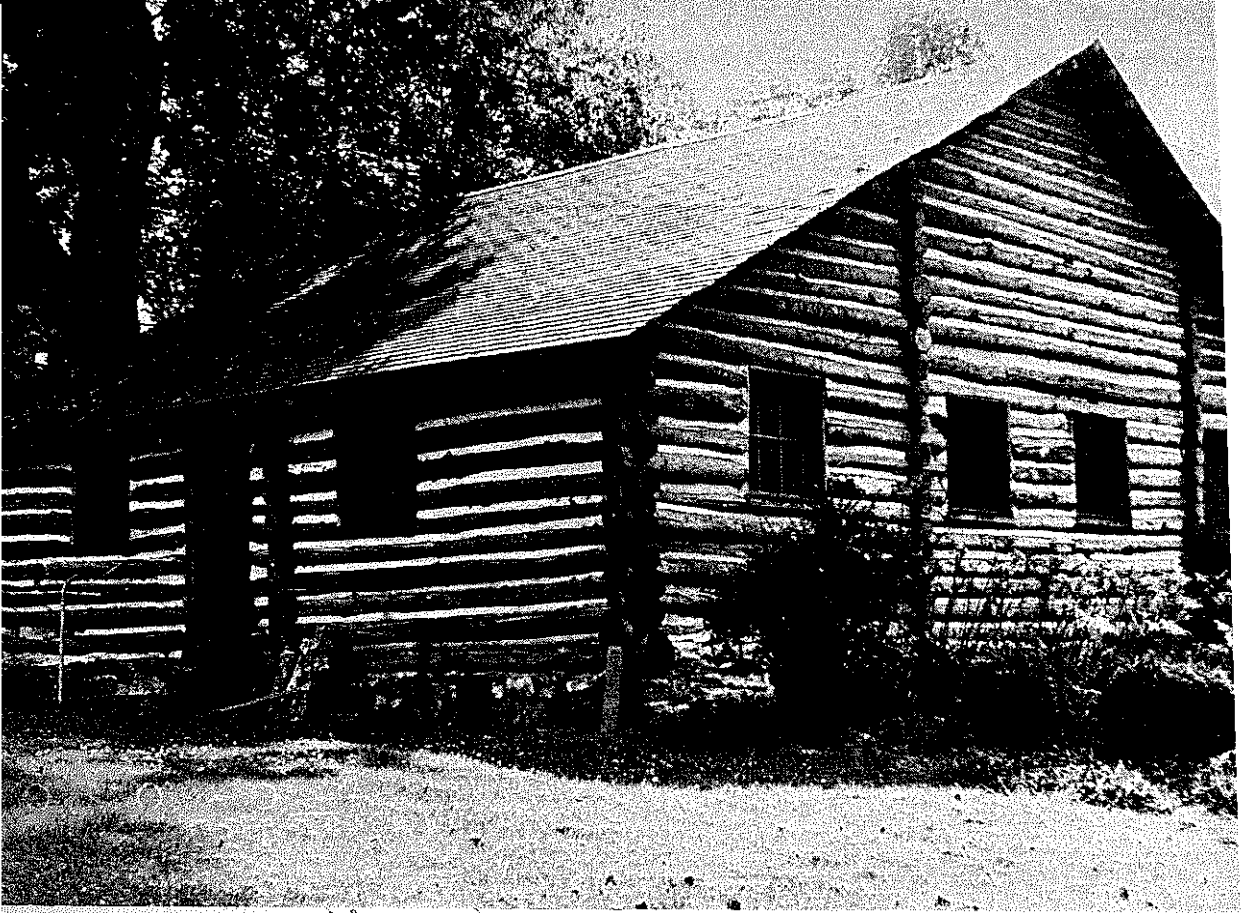
PLATE 126 The Happ'n'so house has pole laths that are really only two feet long and serve only to help support the gable logs and the overhang. The house has a full set of pole rafters.
