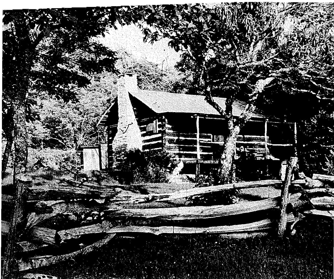
PLATE 39 This building near Highlands, North Carolina, shows why one might still take the time to build a log cabin.
