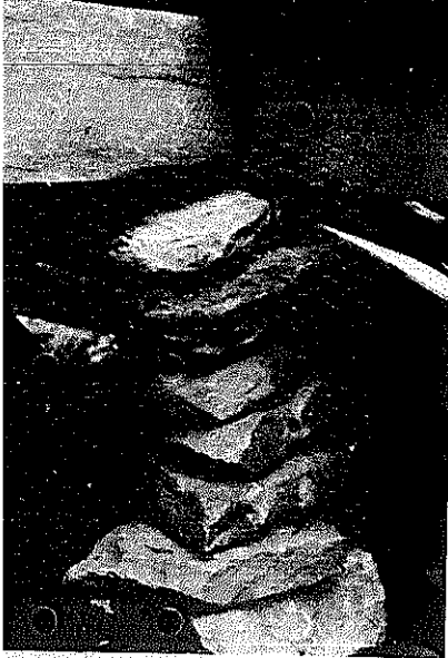
PLATE 44 A foundation pillar made of rocks placed atop each other.
