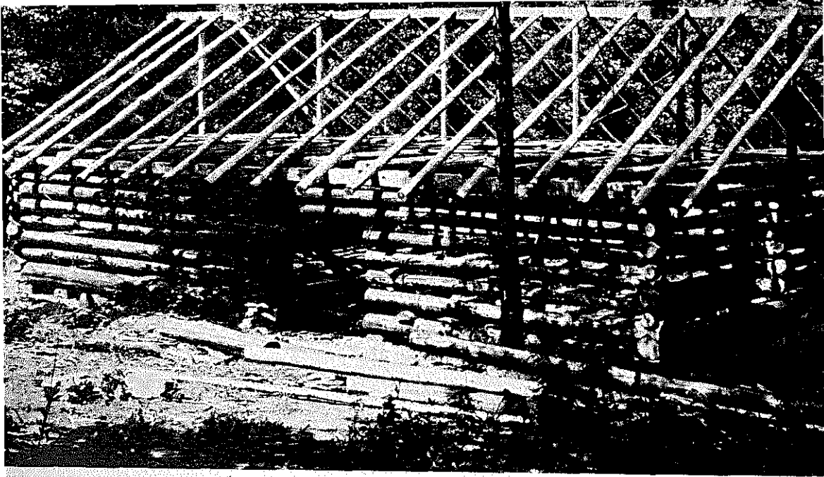
PLATE 128 Roy Thompson's cabin before . . .
