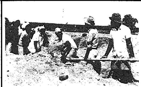
People of Shajiluru village laying plastic water pipes under self-help. The pipes were paid for by the villagers themselves.
