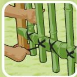
Tie each juncture.
