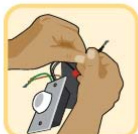
Twist matching wires together.
