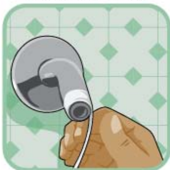
Seal with the pipe tape.
