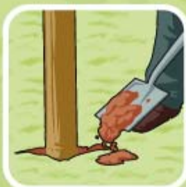
Fill the holes; tamp down.
