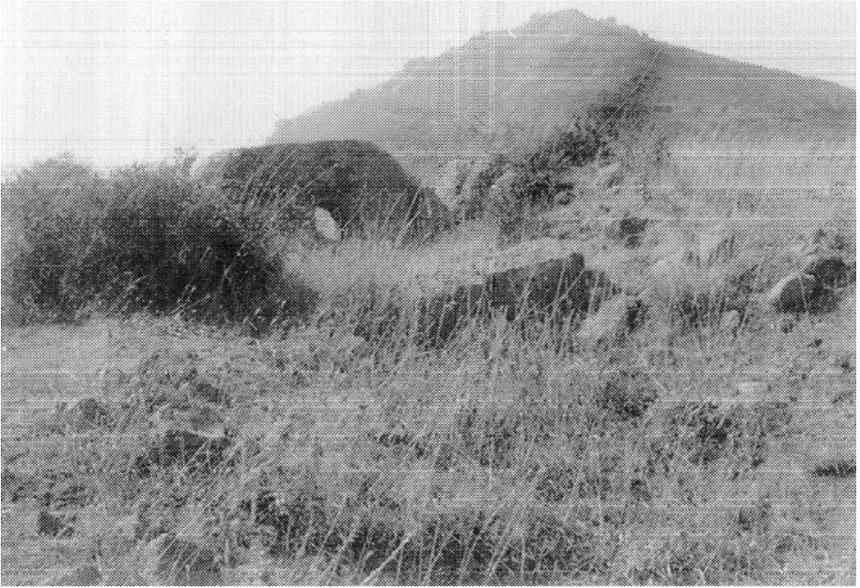
**Figure 22.12.** Largest lockstone of the pressure pipeline at Pergamon, perhaps 2 meters in width, and placed at the top of the hill shown in Fig. 22.13, where the pressure put the greatest strain on the siphon system.
