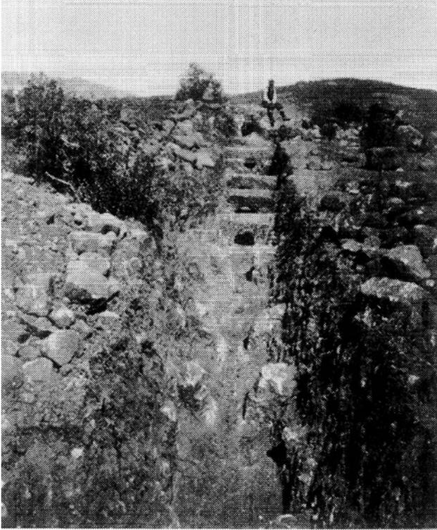
**Figure 22.11.** View of the Hellenistic pressure pipeline north of Pergamon, shown by its lockstones still in situ; the lead pipes have been robbed out but left traces of lead in the soil under the line. This photo was published by H. Graber, in “Die Wasserleitungen von Pergamon,” 1888; he was one of the hydraulic engineers brought in by the early excavators to investigate the water supply of the site. Graber reported finding slivers of lead between the lockstones.
