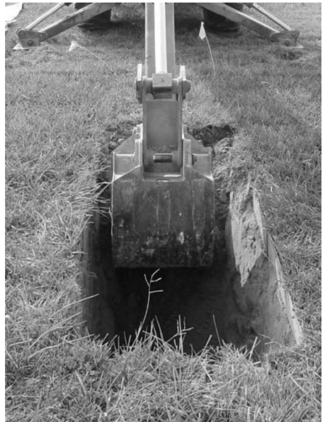
Figure 2. Backhoe digging trench for lysimeter installation.
