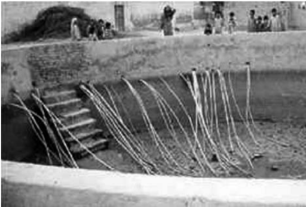
Figure 6. House connections in dry tank.
