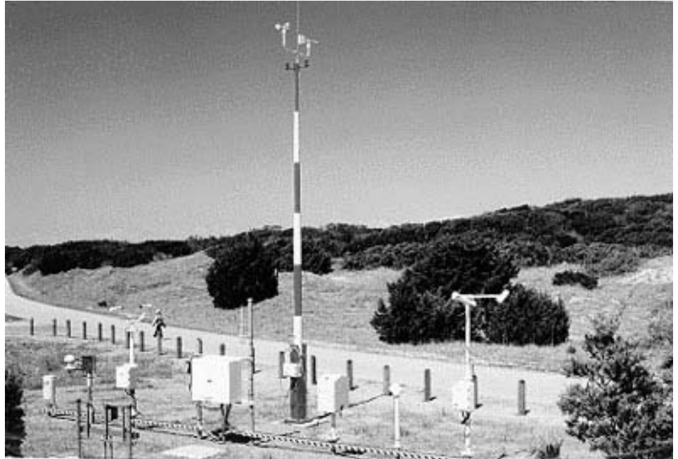
Figure 13. An Automated Surface Observing System (ASOS) installation at Cape Hatteras, North Carolina.
