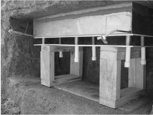
Figure 3. Rectangular cavity excavated in sidewall of the trench with nearly completed lysimeter installation.
