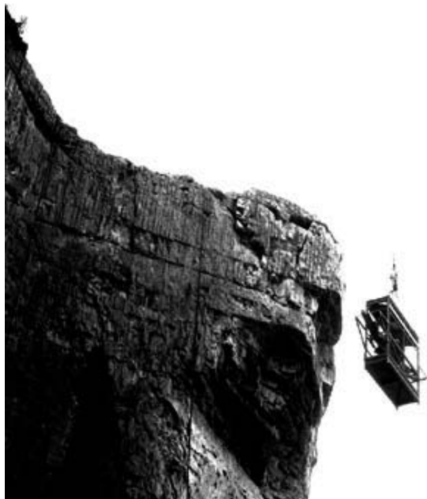
Workers were lowered by cranes, in safety cages, to inspect the face of the falls
