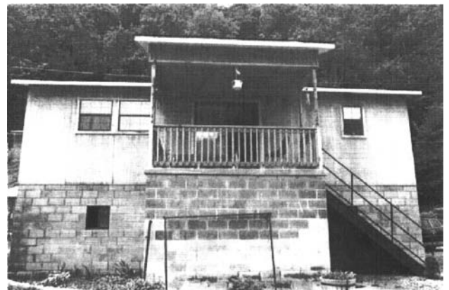
Figure 5. Elevated home in West Virginia is a mitigation success story. Risk is greatly reduced to homes elevated before a flood.
