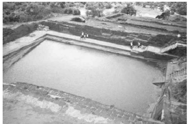
Figure 1. Communal rainwater sotrage.
