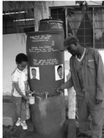
Figure 4. The EnDeCo Institutional Defluoridator. It can be made at any desired capacity, normally in the range 20–160 m 3 for a raw water fluoride of 5 mg/L.
