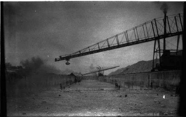
Figure 2. Excavation of the rock section.
