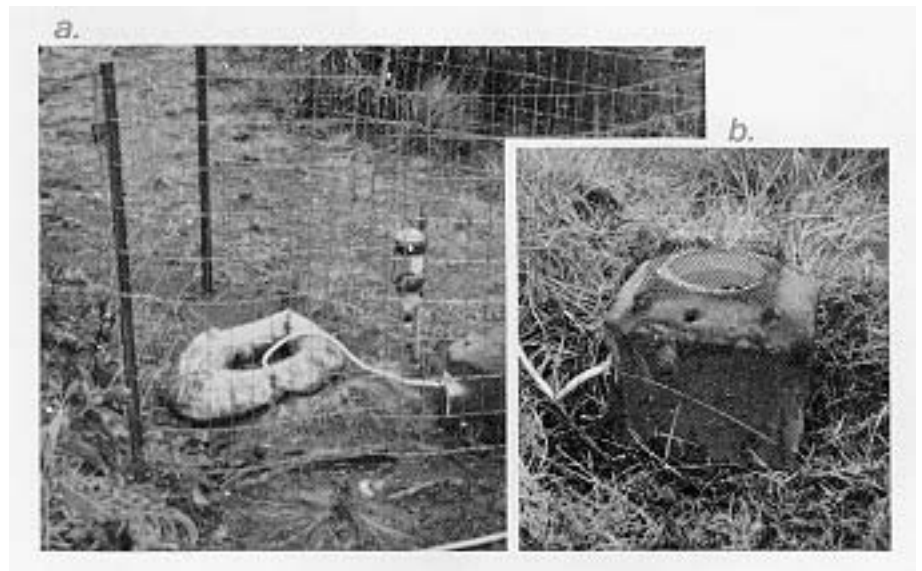
Figure 6. Constant-level pan evaporimeter. a) field installation with inner tube reservoir; b) evaporimeter detail. Note foam insulation around evaporation pan.
