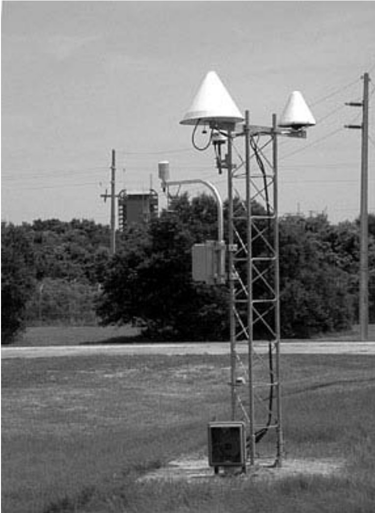
Figure 8. GPS-IPW installation at the U.S. Coast Guard Differential GPS site at Cape Canaveral Air Force Station.
