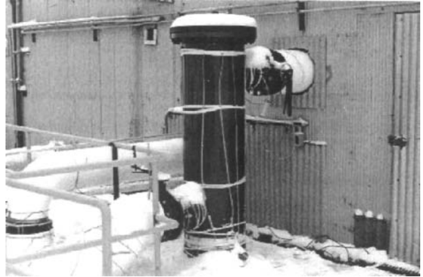
Figure 6. Diagram of industrial setup. Industrial magnetic water treatment system installed at a manufacturing plant on a parallel feed line with a flow rate of 1600 gallons per minute.
