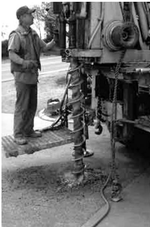
Figure 2. Close-up of a hollow-stem auger rig (Courtesy of Joe Ryan, University of Colorado).
