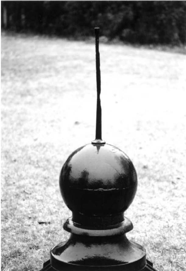
Figure 1. Ventilator/Lightning Rod from Gay Head Lighthouse wick 1900, Martha’s Vineyard, Massachusetts (photograph courtesy of William Waterway).
