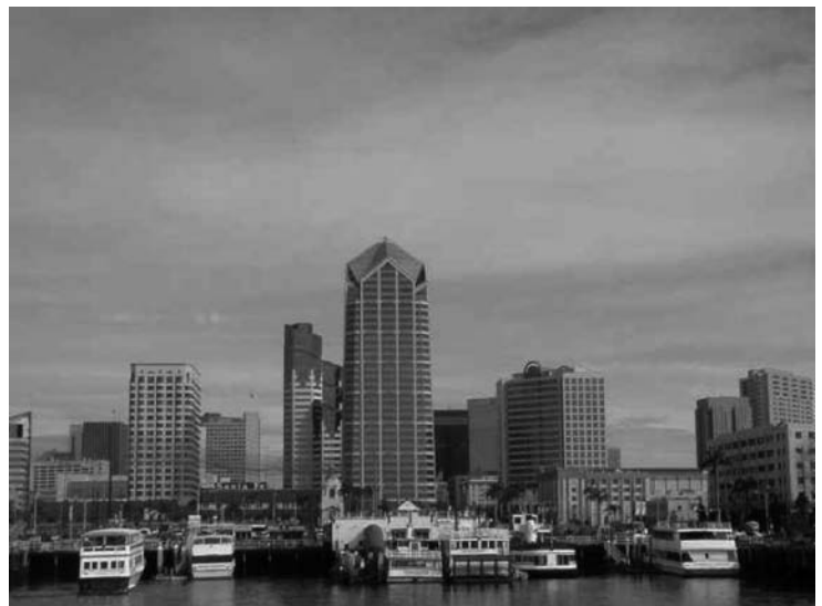
Figure 1. San Diego uses EDR technology to produce low salinity irrigation water from reclaimed municipal wastewater.
