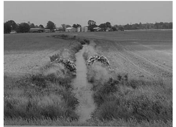
Figure 2. Overgrown constructed ditch draining farm field.
