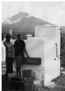
Figure 4. The EnDeCo Institutional Defluoridator. It can be made at any desired capacity, normally in the range 20–160 m 3 for a raw water fluoride of 5 mg/L.
