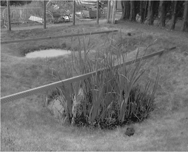
Figure 1. Experimental ponds treating road runoff in Scotland.
