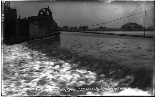
Figure 3. A total of 4250 cubit feet per second passes over the Bear Trap Dam.
