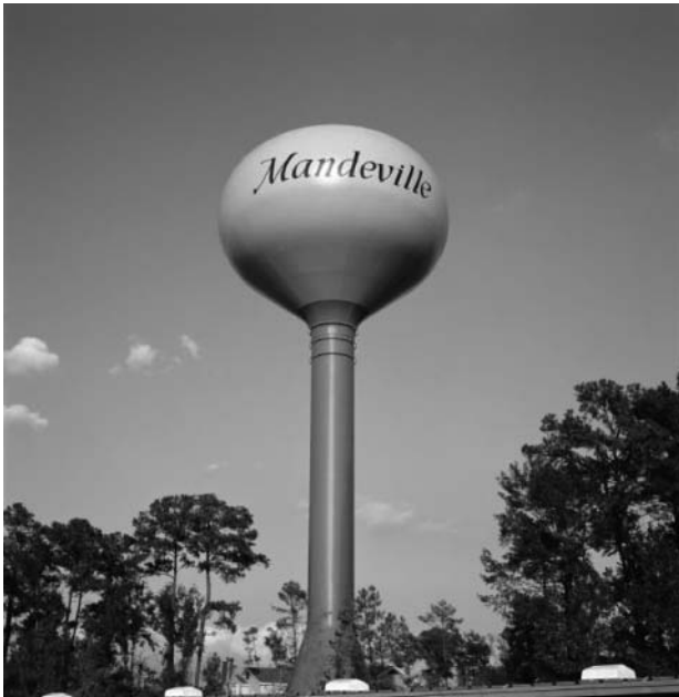
Figure 4. Pedesphere elevated storage tank (Source: Caldwell Tank, Inc.).
