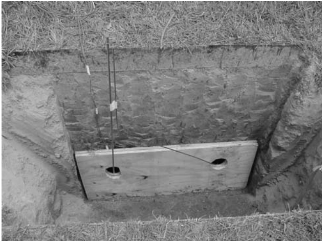
Figure 4. Complete lysimeter installation with cavity protected from damage upon backfilling with treat plywood.
