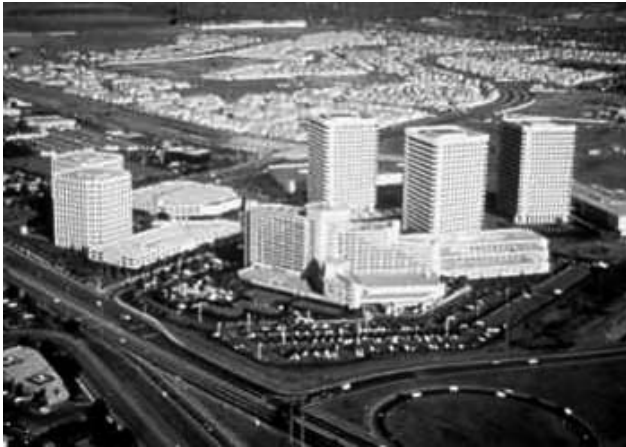
The Irvine Ranch Water District provides recycled water for toilet flushing in high rise buildings in Irvine, California. For new buildings over seven stories, the additional cost of providing a dual system added only 9% to the cost of plumbing.
