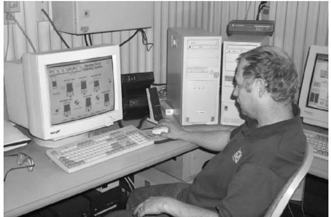
John Barkey, plant operator for Martin's Ferry, Ohio, inspects the water levels of the system's storage tanks from his desk
