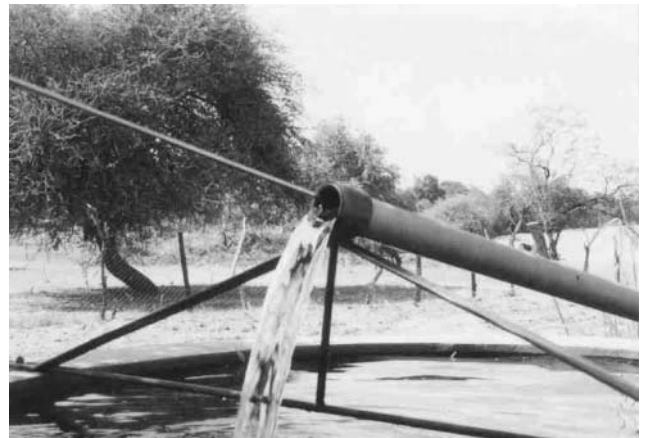
Figure 4. Small-scale, hand pump sand-abstraction scheme.
