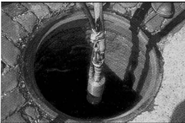
Figure 8. Application of one-coat cementitious structural liner.
