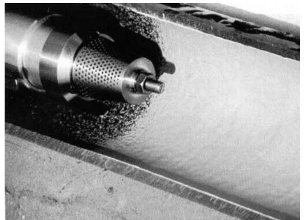
Figure 6. Application of epoxy resin lining.
