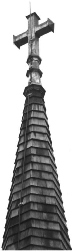
Figure 3. A cross with lightning rod attached. Location: Town of Oak Bluffs on Martha's Vineyard, Massachusetts (photograph courtesy of William Waterway).
