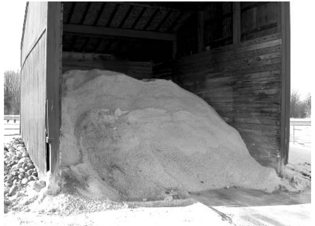
Figure 1. A road salt storage facility open to the elements that can increase runoff during heavy rain effects. This facility is on a parking lot near Lansing, MI (photo by M.E. Benbow).
