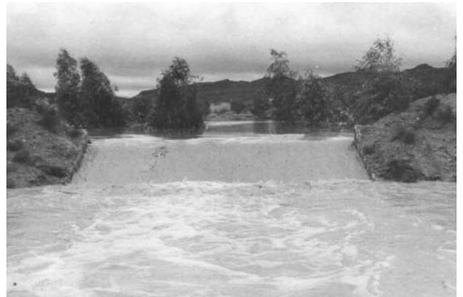
Figure 2. A spillway along a contour dike during operation (Ghareh Baygon Flood Spreading Station, Fars Province, Iran).
