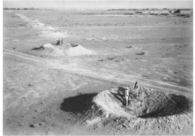
Figure 2. A top view of a qanat during construction.
