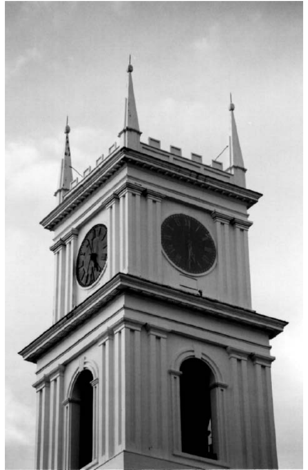
Figure 4. Four lightning rods on top of old Whaling Church, Edgartown, Massachusetts (photograph courtesy of William Waterway).
