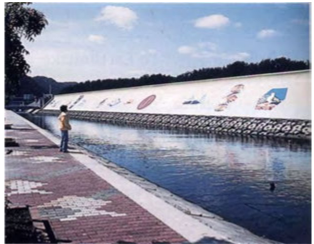
Figure 13.22 Tsunami barrier in the town of Taro, Japan. [Courtesy of Taro, Japan.]
