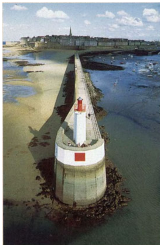
Construction of groins along a shore to control erosion of a beach may result in erosion downcurrent of the groin and loss of parts of the beach ( right of groin ) while sand piles up on the other side ( left of groin ). Longshore current flows from left to right. [Philip Plisson/Explorer.]
