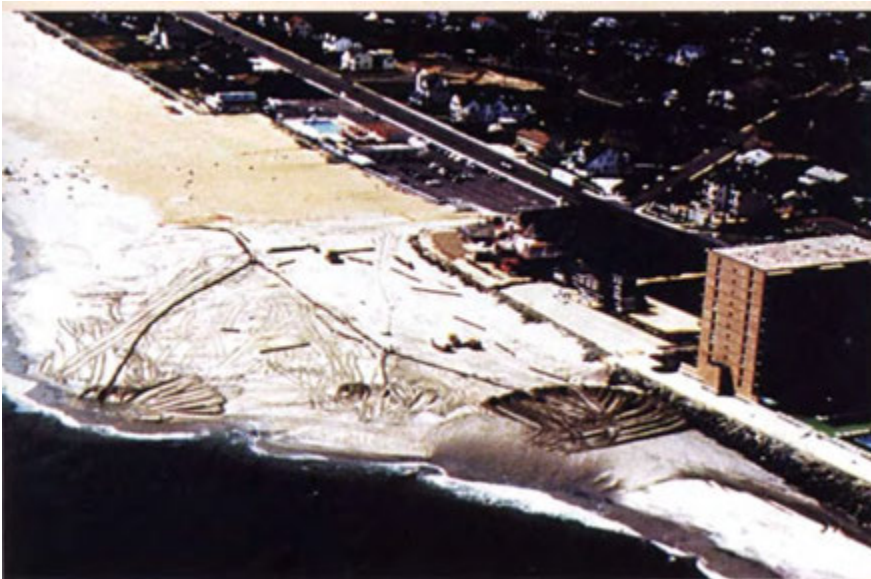
Beach-fill placement at the southern end of Monmouth Beach, Monmouth County, New Jersey. This erosion control project by the U.S. Army Corps of Engineers includes periodic nourishment of the restored beaches on a 6-year cycle for a period of 50 years. [U.S. Army Corps of Engineers, New York District.]
