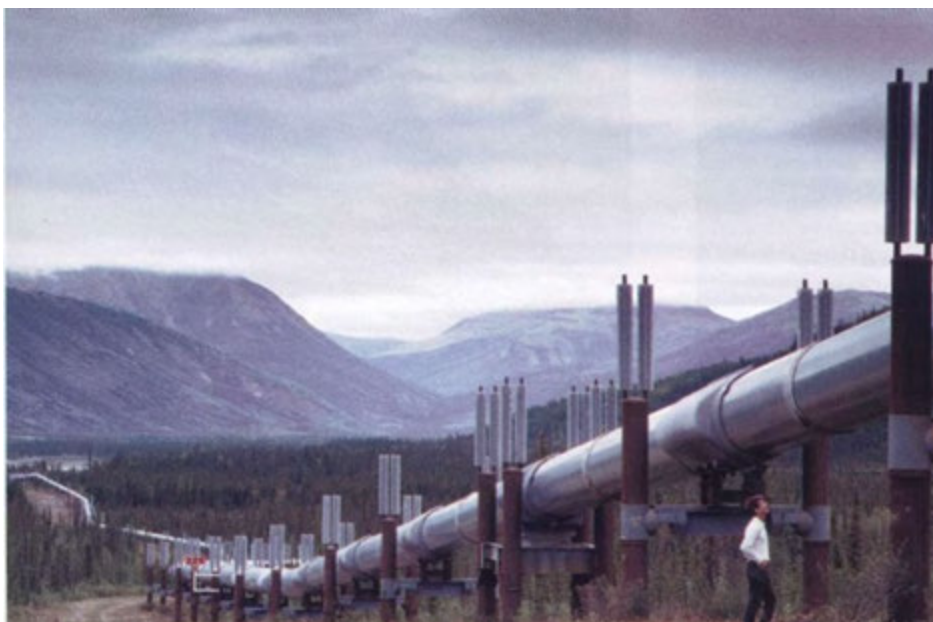
Figure 21.20 Along its 1300-km route from Prudhoe Bay to Valdez, the Alaska oil pipeline crosses 675 km of permafrost, perched on specially designed vertical supports. Because thawing of the permafrost would cause the supports to become unstable, they are outfitted with heat pumps designed to keep the ground around them frozen. The heat pumps contain anhydrous ammonia that vaporizes below ground and rises and condenses above ground, discharging heat through the two aluminum radiators atop each of the vertical supports. [Galen Rowell/Corbis.]
