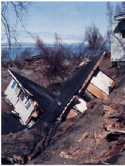
Figure 16.16 Landslide at Turnagain Heights, Alaska, triggered by the earthquake of 1964. [Steve McCutcheon/Alaska Pictorial Service.]
