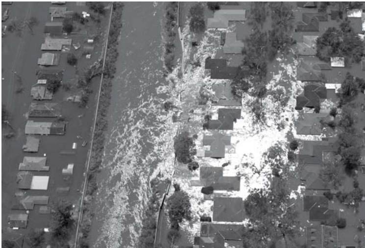
New Orleans: water finally gets the better of engineering in 2005's Hurricane Katrina disaster
