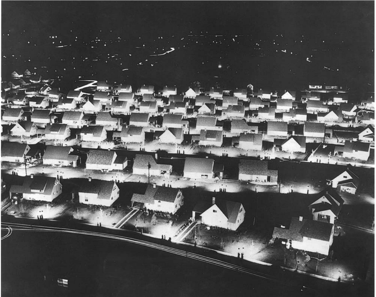
LEVITTOWN — ONE OF THE FIRST POSTWAR SUBURBS The first houses in Levittown in New York in 1947 cost buyers as little as $8000 because they were built with mass-production techniques developed by the U.S. armed services in World War II. As the suburb grew, the builder introduced models with variations that reduced the uniform appearance, although there were still only two basic models in the early 1950s.
