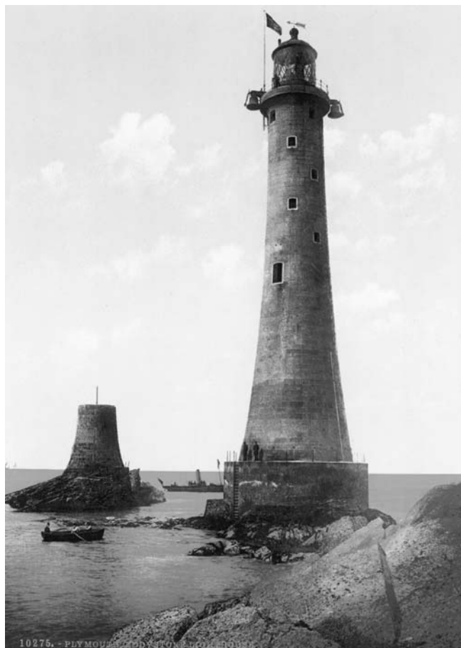
THE PRESENT EDDYSTONE LIGHT The dangerous Eddystone rocks off Plymouth, England, were the site of the first lighthouse to be built in the open sea. The present light completed in 1882, here seen at low tide, reveals the cylinder at the base. Above that the design is still remarkably similar to the one Smeaton used in the 18th century, although the new design by John Douglass is built on a different rock from the previous Smeaton lighthouse.
