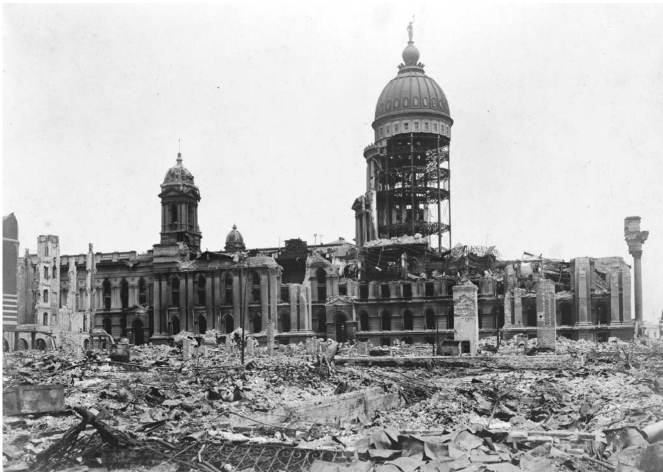
SAN FRANCISCO CITY HALL AFTER 1906 EARTHQUAKE Although not the largest earthquake in U.S. history, the 1906 quake along the San Andreas Fault was the most destructive. The earthquake was felt strongly from Coos Bay, Oregon, to Los Angeles in southern California. In San Francisco itself much of the damage was caused by four days of fire that followed the earthquake.
