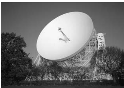
THE 76-M (250-FT) LOVELL TELESCOPE AT JODRELL BANK When the Lovell Telescope was completed in 1957 it was the largest steerable radio telescope ever built (and is still the third largest). Not only has the Lovell Telescope been at the forefront of radio astronomy, but it also has frequently been pressed into service for receipt of faint communications from satellites and space probes, starting with Sputnik I.
