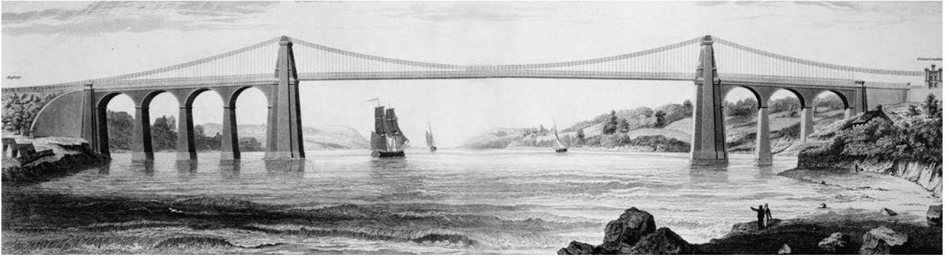
TELFORD'S BRIDGE OVER MENAI STRAITS The first major suspension bridge took six years to build and was a record 176 m (579 feet) in length. The roadway, suspended from a chain of wrought-iron links, had to be 30 m (100 ft) above sea level to permit tall sailing ships to pass under it. The bridge still stands near Anglesey, Wales.
