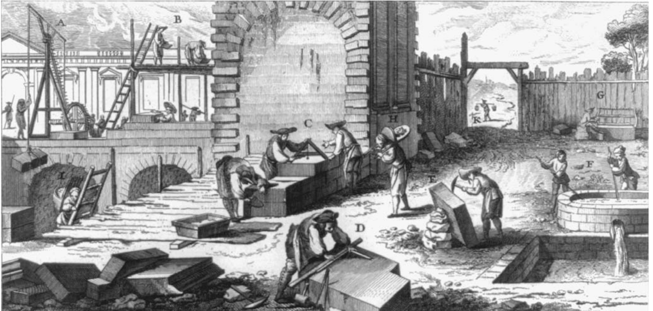
CRAFT OF MASONRY FROM DIDEROT'S ENCYCLOPÉDIE The subtitle of the Encyclopédie is "a rational dictionary of science, arts, and crafts." Today it is especially valued by historians for its 11 volumes of illustrations, which show 18th century crafts, such as cutting and laying stone, in detail.
