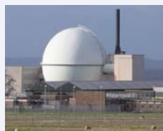
NUCLEAR POWER STATION
