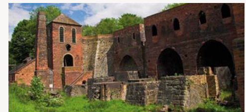
BLAST FURNACE IN IRONBRIDGE, ENGLAND
