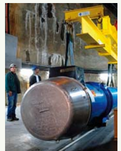
MAGNET BEING FITTED IN THE LHC
