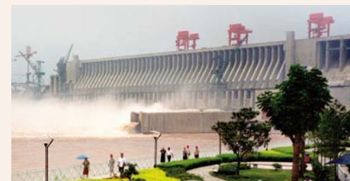
THREE GORGES DAM, CHINA
