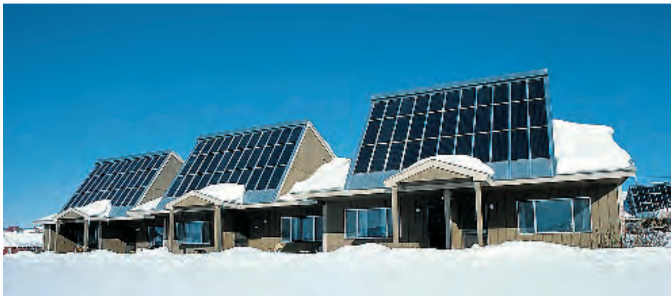
Figure 16 The roofs of these houses are covered with solar cells, which use sunlight to produce electricity. On sunny days, the people living in these homes help preserve natural resources by using electricity generated by the Sun instead of a power plant.
