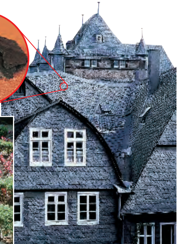
The roof of this house is made of slate, a foliated metamorphic rock.
