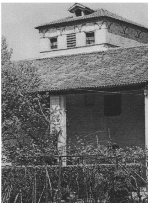
Figure 6: Pozzoleone (Italy), Tower of the Villa Gonzato.
