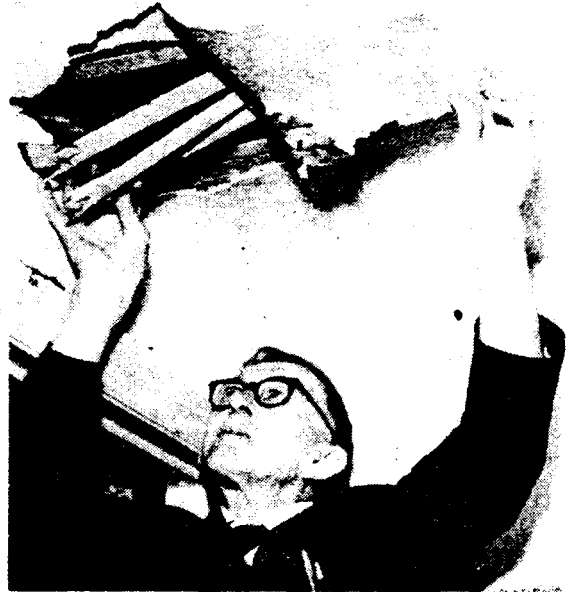
Mr. Frank Walker inspects the damage to his ceiling.
