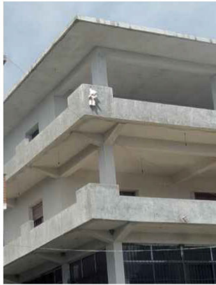
ABOVE: Teddy on a half-finished building, Belesh;
