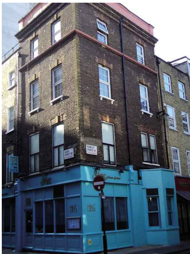
LEFT: The house at 36 Greek Street, as it looks today.
