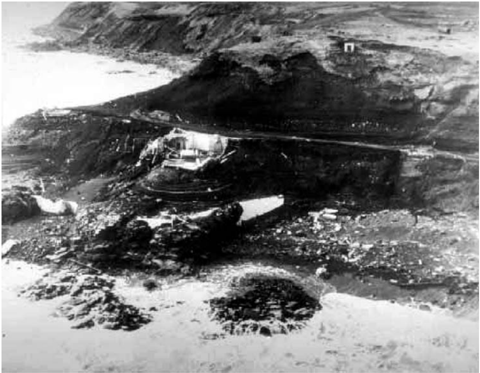
Figure 2.9. The remains of the Scotch Cap lighthouse, Unimak Island, Alaska, following the April 1, 1946 tsunami. A Coast Guard station, situated at the top of the cliff 32 m above sea level, was also destroyed. Five men in the lighthouse at the time perished. Source: United States Department of Commerce, National Geophysical Data Center.
