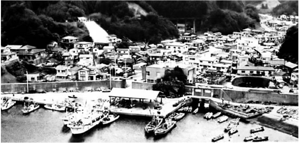
Figure 9.9. Ryoishi, a typical town along the Sanriku coast of Japan protected against tsunami by 4.5 m high walls. These walls are now common around the Japanese coast; however, they do not offer protection against tsunami having historical run-ups. Source: Fukuchi and Mitsuhashi (1983).
