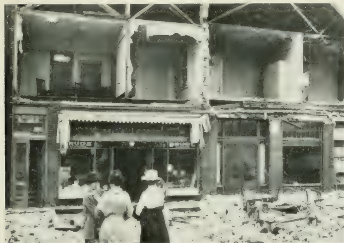
FIGURE 3. Damage to weak masonry, Inglewood, 1920. Separation of bricks was due to weak mortar. Seis. Soc. Amer., Bull., vol. 10, plate 8. Photo by Los Angeles Times.
