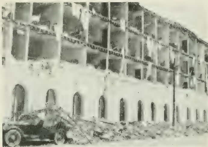
FIGURE 4. Damage to weak masonry, frame structure with brick veneer, Santa Barbara, 1925. Seis. Soc. Amer., Bull., vol. 15, plate 30.
