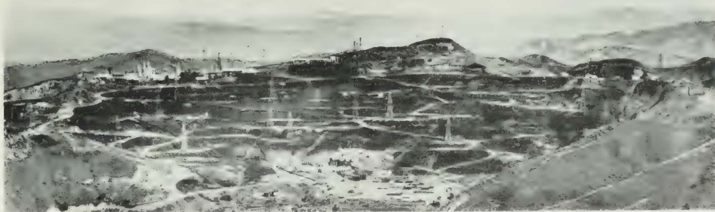
Fig. 21. Landslide in Ventura Avenue oil field. Surface of slide covering approximately 160 acres, has been contoured and oiled.
