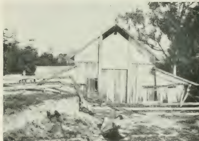
FIGURE 8. Barn not seriously damaged, although fault trace passed under one corner, 1906. Near Olema. California Earthquake Commission Report.
