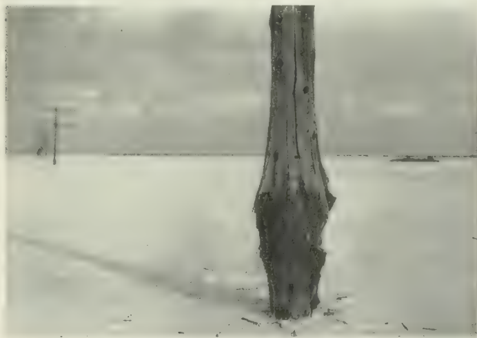
FIGURE 6. The effects of crystallizing salt on telegraph poles, in the salt flat east of Wendover, Utah.
