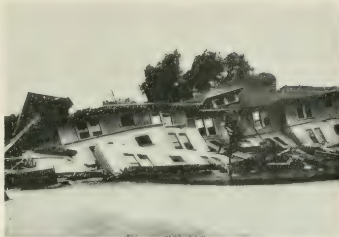
FIGURE 7. Collapse of weak frame structure. Hotel in San Jose, 1906. California Earthquake Commission Report.
