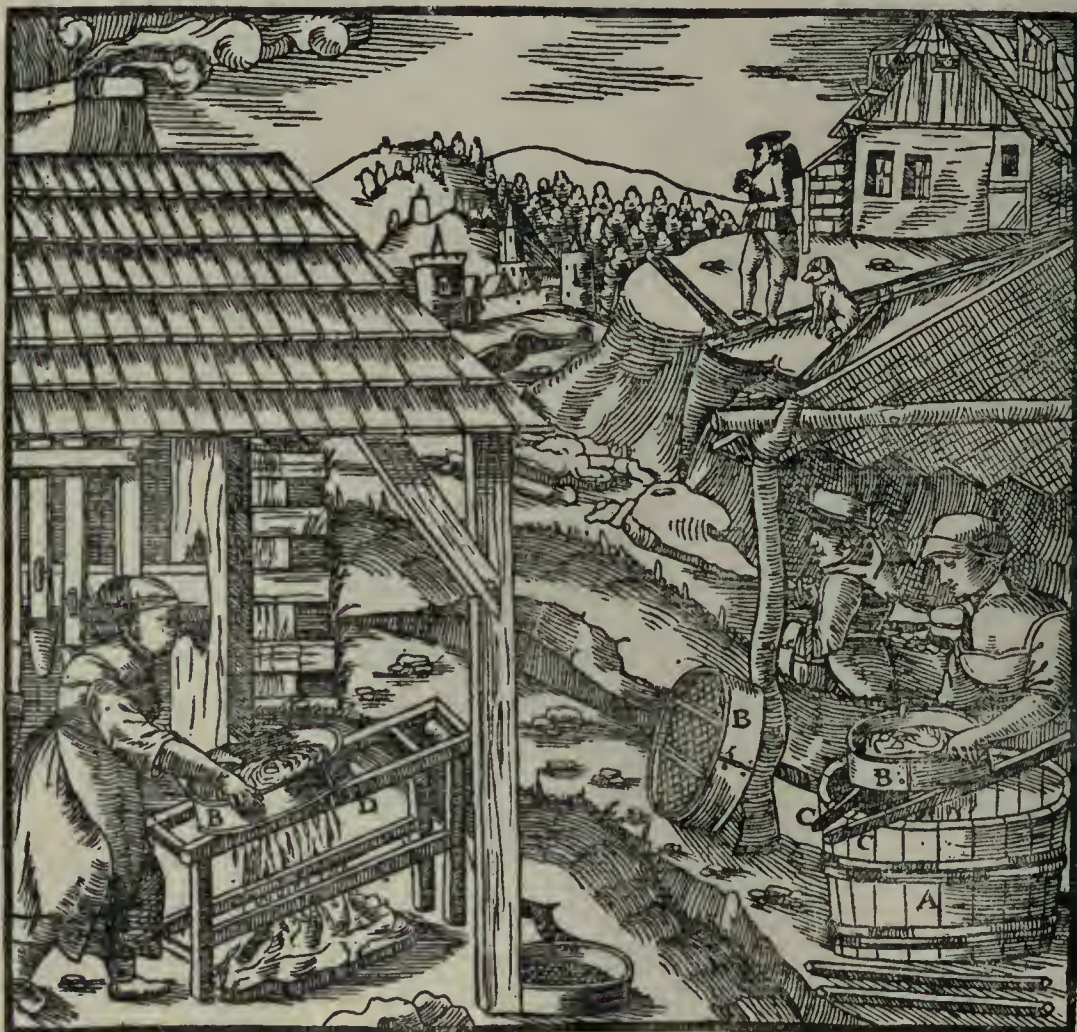
A—TUB. B—SIEVE. C—RODS. D—BENCH-FRAME.
