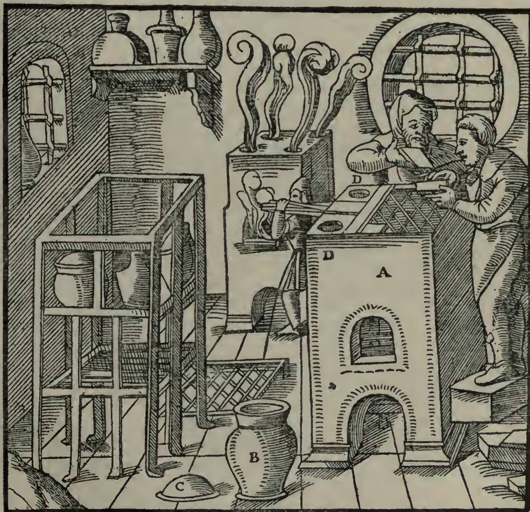
A—FURNACE. B—POT. C—LID. D—AIR-HOLES.
