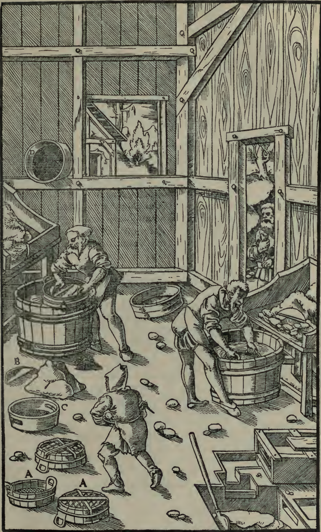
A—FINE SIEVES. B—LIMP. C—FINER SIEVE. D—FINEST SIEVE
