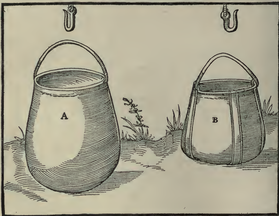
A—WATER-BAG WHICH TAKES IN WATER BY ITSELF. B—WATER-BAG INTO WHICH WATER POURS WHEN IT IS PUSHED WITH A SHOVEL.
