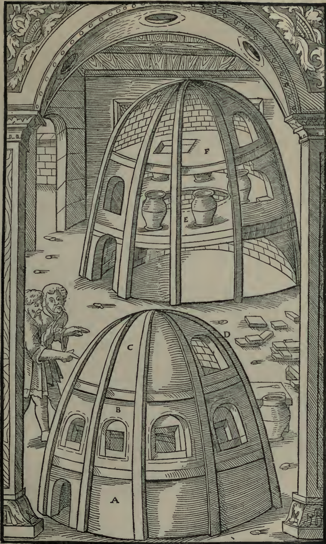
A—LOWER CHAMBER OF THE OTHER SECOND FURNACE. B—MIDDLE ONE. C—UPPER ONE. D—ITS OPENING. E—ROUND OPENING. F—RECTANGULAR OPENING.
