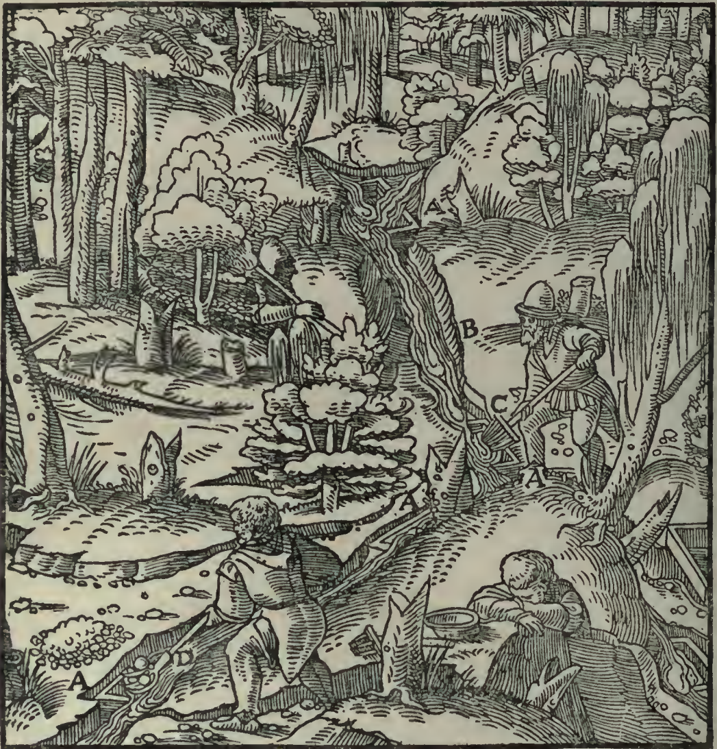
A—PITS. B—TORRENT. C—SEVEN-PRONGED FORK. D—SHOVEL.
