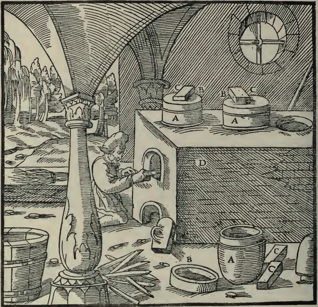
A—POTS. B—LIDS. C—STONES. D—FURNACE.
