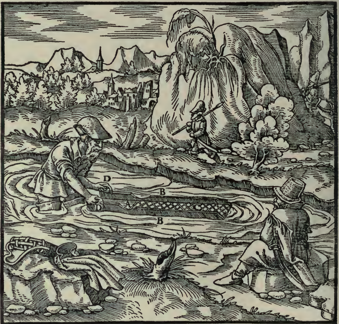
A—PLANK. B—SIDE-BOARDS. C—IRON WIRE. D—HANDLES.
