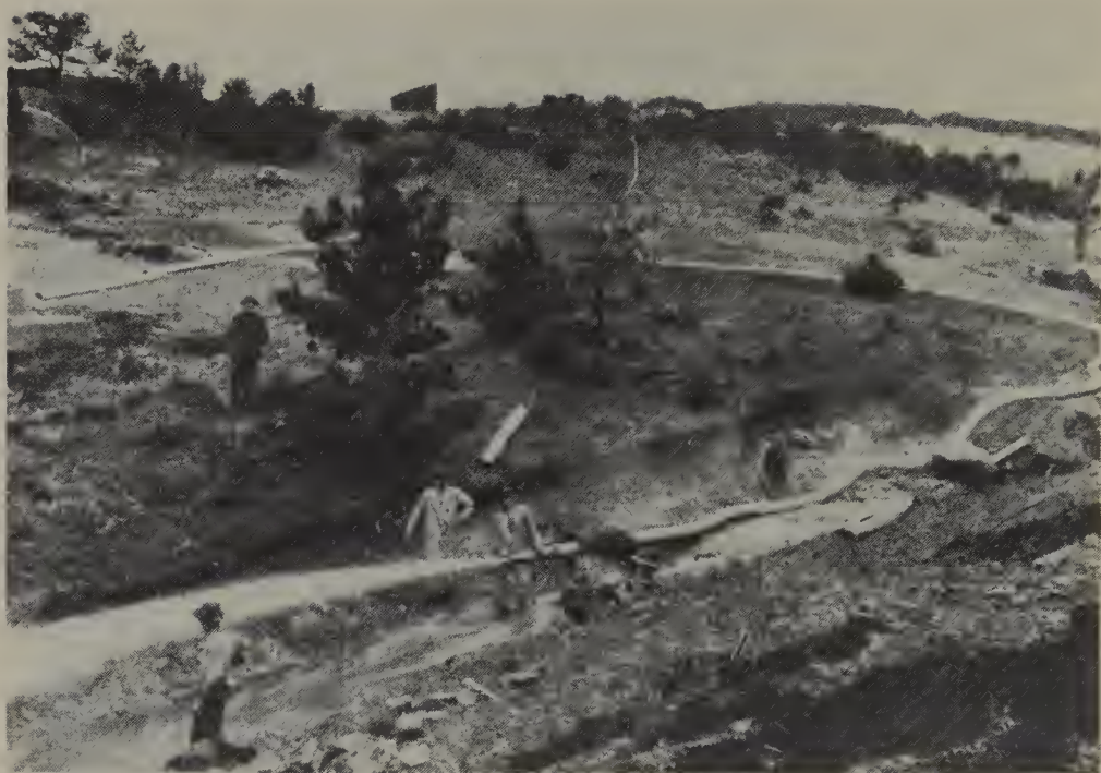
The earliest known photograph of mining at the Yogo dike, taken about 1897. In this hydraulicking operation, the high-pressure hose is used to wash away the weathered surface dike rock into sluice boxes. The trench in which the hose lies is the dike itself. Water was brought by a ditch and flume system from upper Yogo Creek to the top of the hill in the background. Water pressure was gained by the 150-foot "head," or drop in elevation from the hill to the dike.
