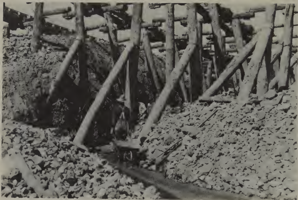
The weathering heaps. Newly mined ore in tiny ore cars was pushed along rails atop the trestles, then dumped into the weathering heaps. Note that the "floor" is timbered to minimize the sapphire loss. In several months, the large pieces of dike rock in these heaps will have deteriorated into a clay-like material suitable for washing.
