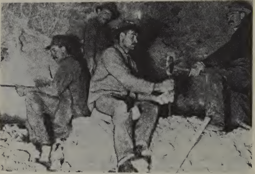
Miners at the English Mine at work in the very early 1900s. The two miners on the right are using an out-dated hand drilling technique known as double-jacking; the miner on the left holds the drill steel while his partner swings away with an eight-pound sledge. The holes were then loaded with light charges of dynamite to blast the solid dike rock loose.
