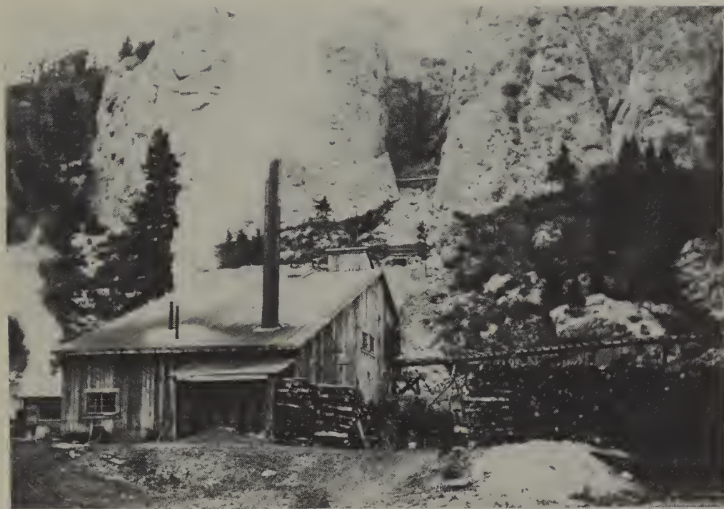
The American Mine mill in Yogo Gulch. Built in 1905 for a cost of $30,000, the mill was able to treat about 100 tons per day. It was last used in 1913 and was finally torn down in the early 1950s. The cleft in the limestone cliffs is the Yogo dike. Natural water erosion had worn away the dike rock leaving only the walls of Madison limestone in place.
