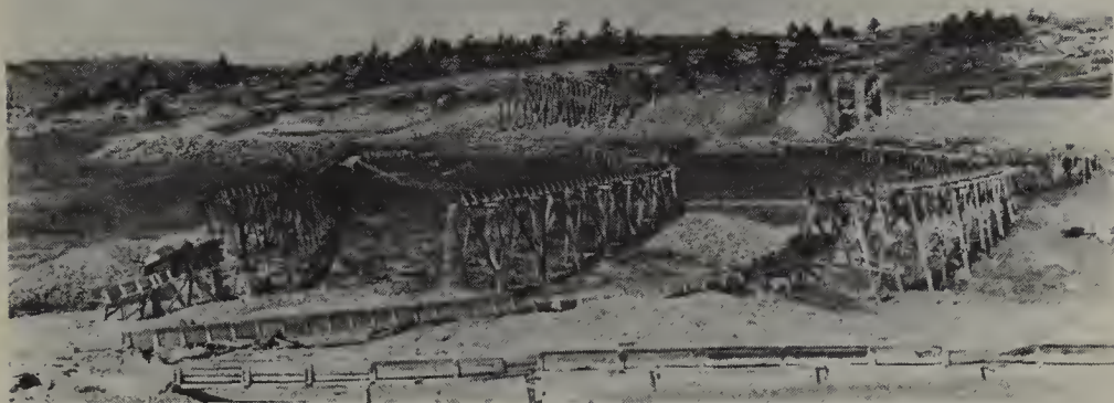
Part of the weathering heaps and system of trestles at the English Mine. This photograph, probably taken about 1906, preceded the installation of timber weathering floors.
