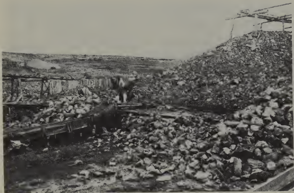
One of the many weathering heaps at the English Mine. Note the trestle at upper right. The trestles were quickly disassembled and moved to new locations as needed to spread the ore over a greater area for maximum exposure to the elements.
