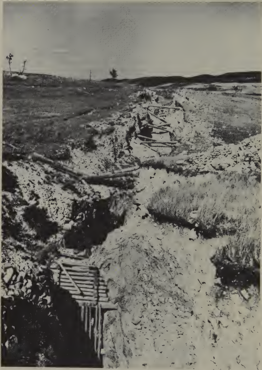
Early surface workings at the Yogo dike. The timbers, or stulls, were used for ground support and to prevent loose rock from falling on the miners below.
