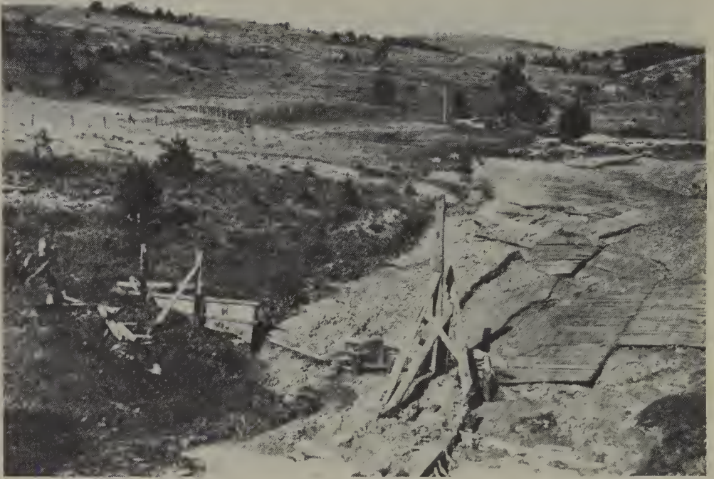
The aftermath of the cloudburst and flooding that occurred on July 26, 1923. This photograph, taken shortly after the disaster, shows the severe damage done to holding dams and weathering floors that effectively terminated production at the English Mine.
