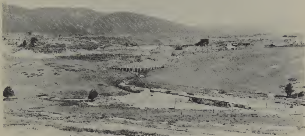
A general view of the English Mine about 1914. The large building is the shaft house which is surrounded by trestles, weathering heaps and tailings dams.
