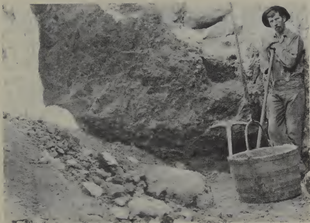
A Yogo miner stands alongside the "sinking bucket" in the first shaft ever sunk into the dike. In this photograph, taken about 1899, the shaft is only about ten feet deep. Eventually, the English Mine underground workings would reach a depth of over 250 feet. Although a steam hoist would be installed as the workings progressed deeper, the English Mine never brought in modern mining equipment.
