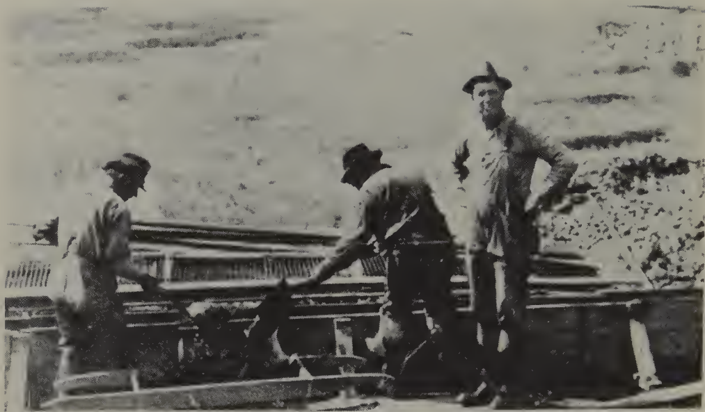
Workmen cleaning a sluice box. The fence-like device behind the workmen are metal riffles which have been removed from the bottom of the sluice boxes. The riffles act as a trap to retain the heavy sapphires during the washing process. Sapphire recovery at the English Mine was very similar to placer gold recovery methods.
