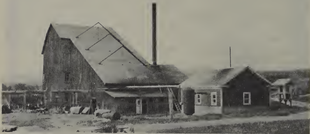
The English Mine shaft house, or head frame, and boiler room. Most of the sapphire production of the English Mine was hoisted to the surface through this building.
