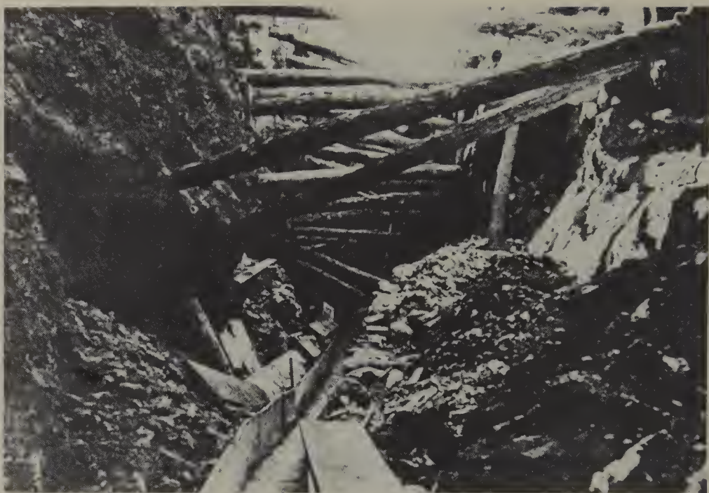
Old English Mine workings. The overhead stulls provide ground support. This section was hydraulically mined and the ruins of the sluice boxes can still be seen.
