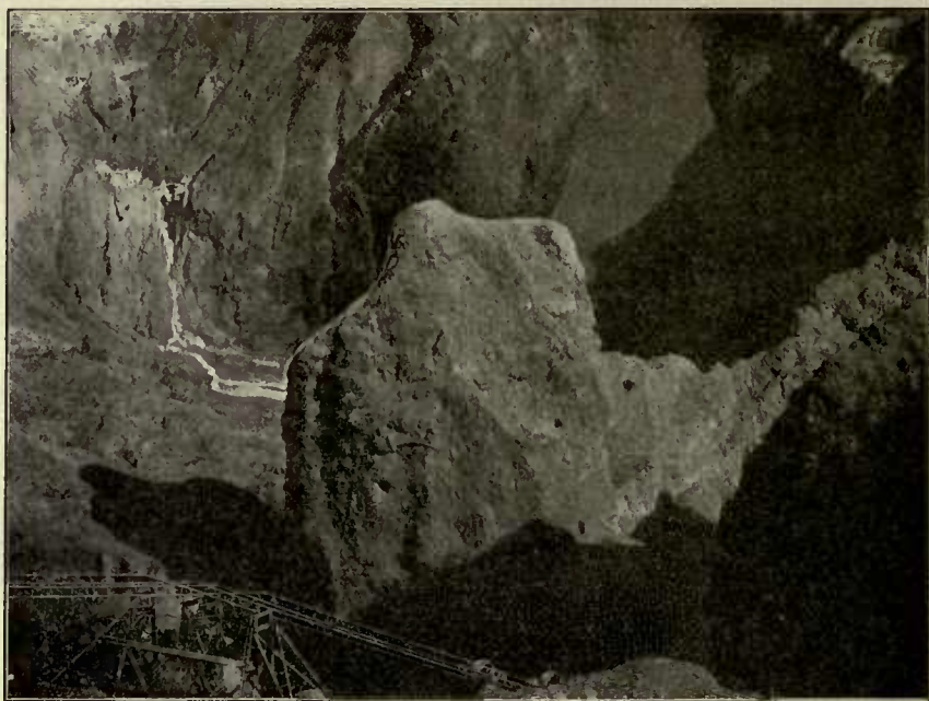
Mount Ararat before Blasting. (Removal of a piece of "Floating Reef," Bultfontein Mine, 1901. It was 150 feet long, 50 feet wide, and 120 feet high. 180 holes were drilled in it and charged with 1050 pounds of No. 1 dynamite.)
