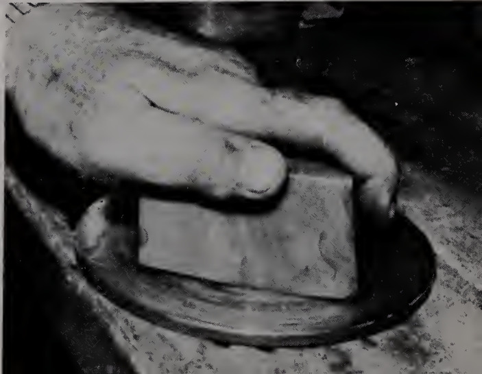
An alternate method is the use of an agate wedae to imprecnate the metal with diamond.
