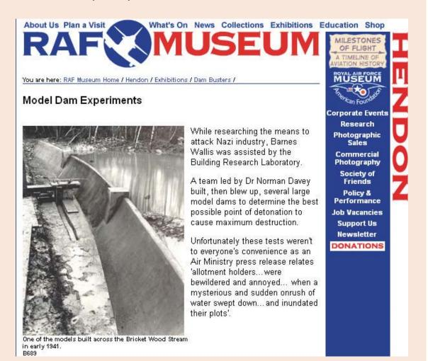
Figure 16.1 An analog model built in 1941 to validate the 'bouncing bomb' ideas of Dr Barnes Wallis in preparation for the successful Royal Air Force assault on German dams in 1943 (Reproduced by permission of Royal Air Force Museum)
