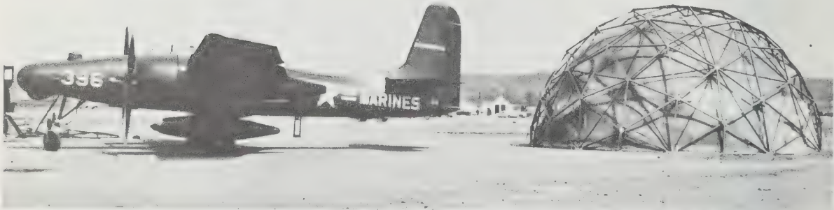
394 At the last assembly of the year, the dome is anchored firmly to the ground. Two 3,000 h.p. driven propellers of an anchored airplane provided day-long slam loads on the dome of 120 m.p.h. winds. The dome never fluttered.
