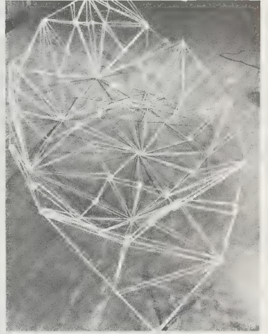
312-316 Thirty-one-great-circle necklace structure of tubular beads and continuous internal cable net, folds up in tight package and unfolds to be tightened finally at its equator into hemispheric dome. The latter is shown in Pentagon Garden, Washington, D.C., February, 1949.
