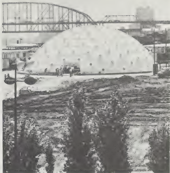
355 One-hundred-foot Geodesic pavilion was built for the mid-continent jubilee, St. Louis, Missouri, on the old fair grounds on the Mississippi River, 1956. This dome now covers the skating rink at Detroit's Northland Shopping Center.
