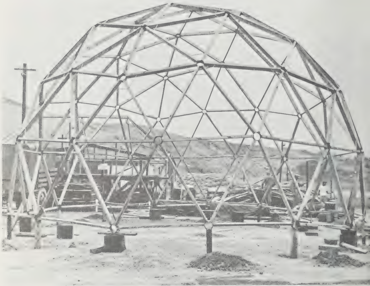
450 Geodesic dome to serve as bachelor officers' quarters, U. S. Air Force, Korea, 1955.
