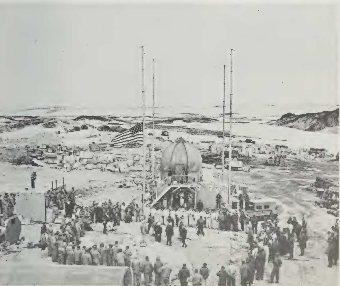
405 One of five Marine Corps Geodesic units, installed at Wilkes Land, Antarctica, in U. S. Geophysical Year base.
