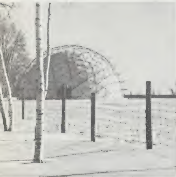
326-328 First large-size (50 feet in diameter) tube and skin structure, erected by the Fuller Research Foundation, Canadian Division, directed and calculated by Fuller's former Institute of Design students, Jeffrey Lindsay and Don Richter, aided by Ted Pope, in Montreal, December, 1950.
