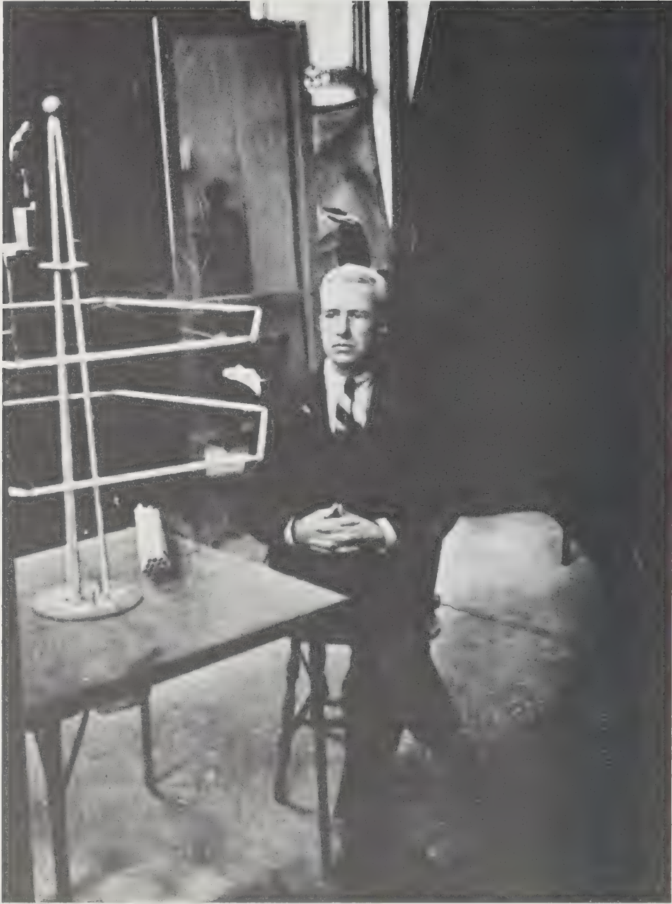
261 Fuller and his first 1927 Tensegrity structure, a mast and double wire-wheel system as seen through the keyhole of a Greenwich Village studio, 1929.
