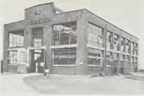
116 The Dynamometer building of the Locomobile plant in Bridgeport, Connecticut, which was taken over by Fuller for development of the prototype Dymaxion cars. (March, 1933)
