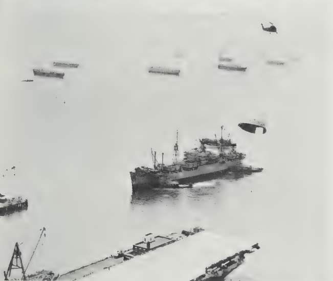
396-400 Geodesic shown first on carrier's flight deck, where helicopter lifts and flies it away at 60 knots to effect beachhead maintenance cover for aircraft.
