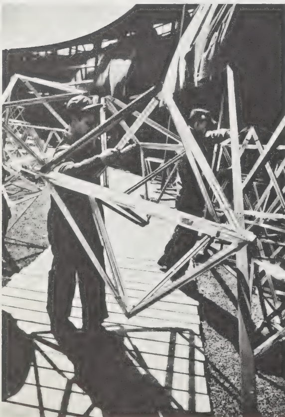
292-297 Four-pound octahedra associated in Octet Truss complex were joined together to form the Ford Motor Company's 93-foot-diameter Rotunda dome, weighing a total of 8½ tons.
