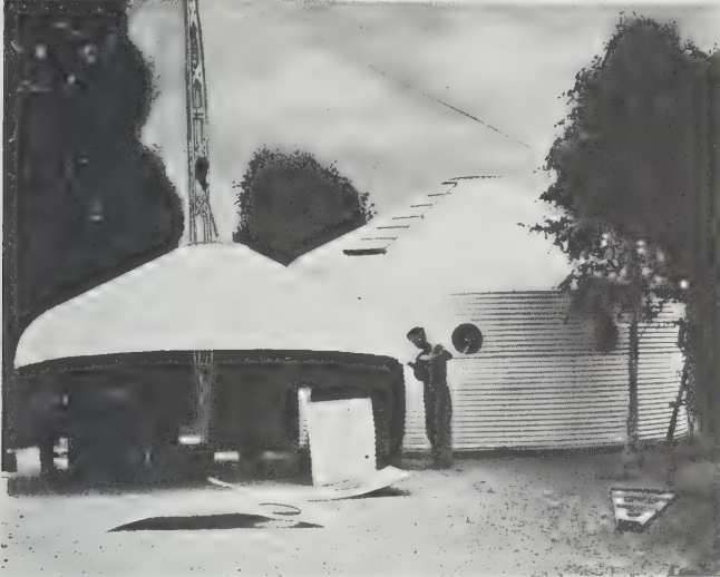
181 Twin Dymaxion Deployment Unit being installed in the garden of the Museum of Modern Art, New York City, in the summer of 1941. Note the metal masts and their integral winching apparatus. These became standard items in the packaged unit delivered to the Armed Services.
