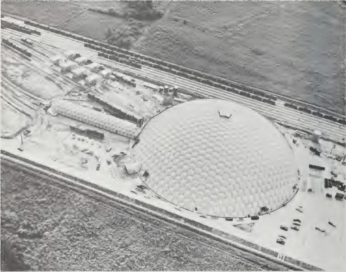
482-483 Exterior and interior of all-steel Union Tank Car Company's Geodesic dome, 384 feet in diameter and 116 feet high. It was opened in Baton Rouge, Louisiana, October, 1958, as car rebuilding plant. At that time it was the largest clear-span enclosure ever built anywhere.
