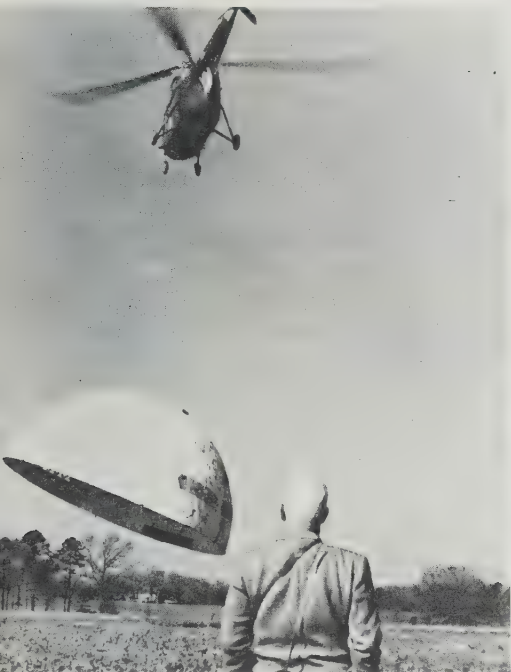
387-388 Fuller witnesses Marine Corps helilift of his 30-foot, wood and plastic Geodesic, at Orphan's Hill, North Carolina, February 1, 1954. Marines flew dome at 50 knots without yaw, and returned to original spot without damage. This event inaugurated the Marine Corps' rigorous investigation and eventual adoption of Geodesic structures.
