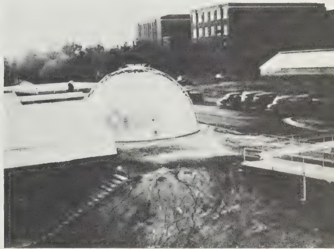
342-343 Thirty-six-foot, transparent Geodesic "Growth House," fabricated by North Carolina State architecture and agricultural science students, 1953. The double-skin dome slid upwardly from its foundation to increase base ventilation through screened accordion opening 18 inches in height.
