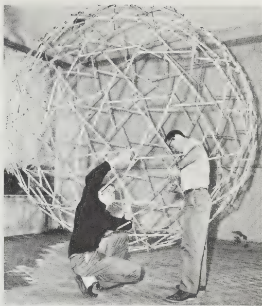
279 University of Oregon students, 1959, with 270-strut Tensegrity, in which every component is identical. In this system, Fuller has broken through to spheroidal systems of unitary modular denominators in frequency magnitudes of infinite series. (Each of the earlier Tensegrity systems required components of several modular dimensions.)
