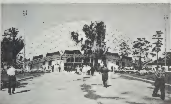
480 Kaiser 200-foot Geodesic, erected as the U. S. main pavilion at the American exchange exhibit in Moscow, 1959.
