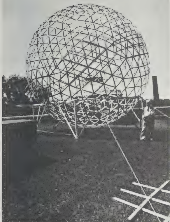
373 Foldable components of Cornell 20-foot Geodesic sphere, 1952.
