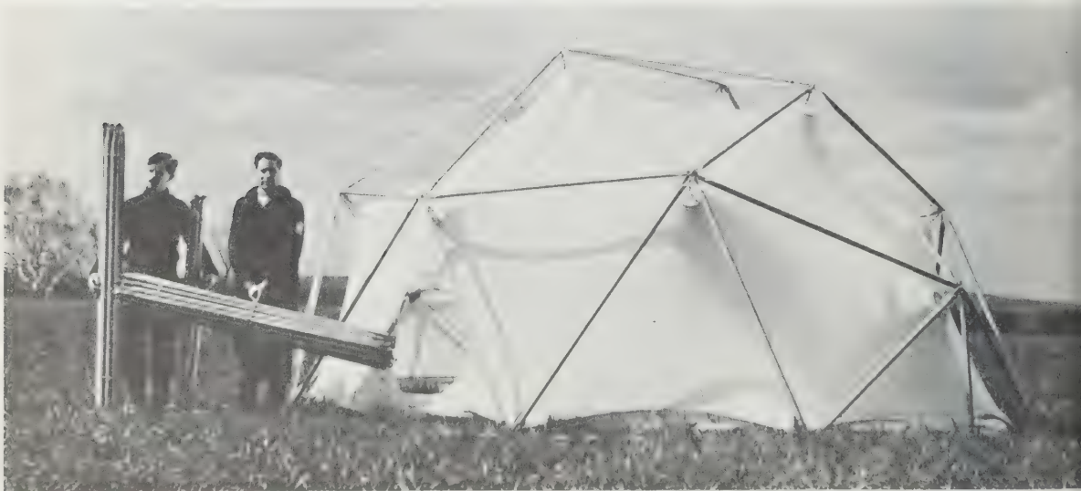
329 Two-frequency Geodesic for Arctic Institute, which went to Baffin's Land in Labrador in 1951, shows hyperbolic parabola (positive-negative curvature) of outwardly tensed "Hypercats" skins which inhibit all flutter.
