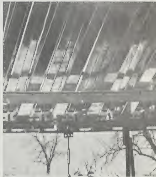
202 Top surface of the floor troughs used for exhaust air conduction from the interior perimeter of the floor area through cove registers. The underside of adjoining floor beams provided the conducting chamber through which incoming cold air was led to central mast. Plywood pie-shaped floor units were superimposed on aluminum floor ribs; they were locked down by "fish-hook hat section" floor joint runner strips, which caught into a trough between the floor ribs, and provided a slide angle into which pie-shaped floor pieces, with beveled edges, were driven like wedged corks. As in the Deployment Unit, Fuller developed a complete floor without using screws, nails, or cement. Result: a completely dry, demountable, muscularly-tight system.
