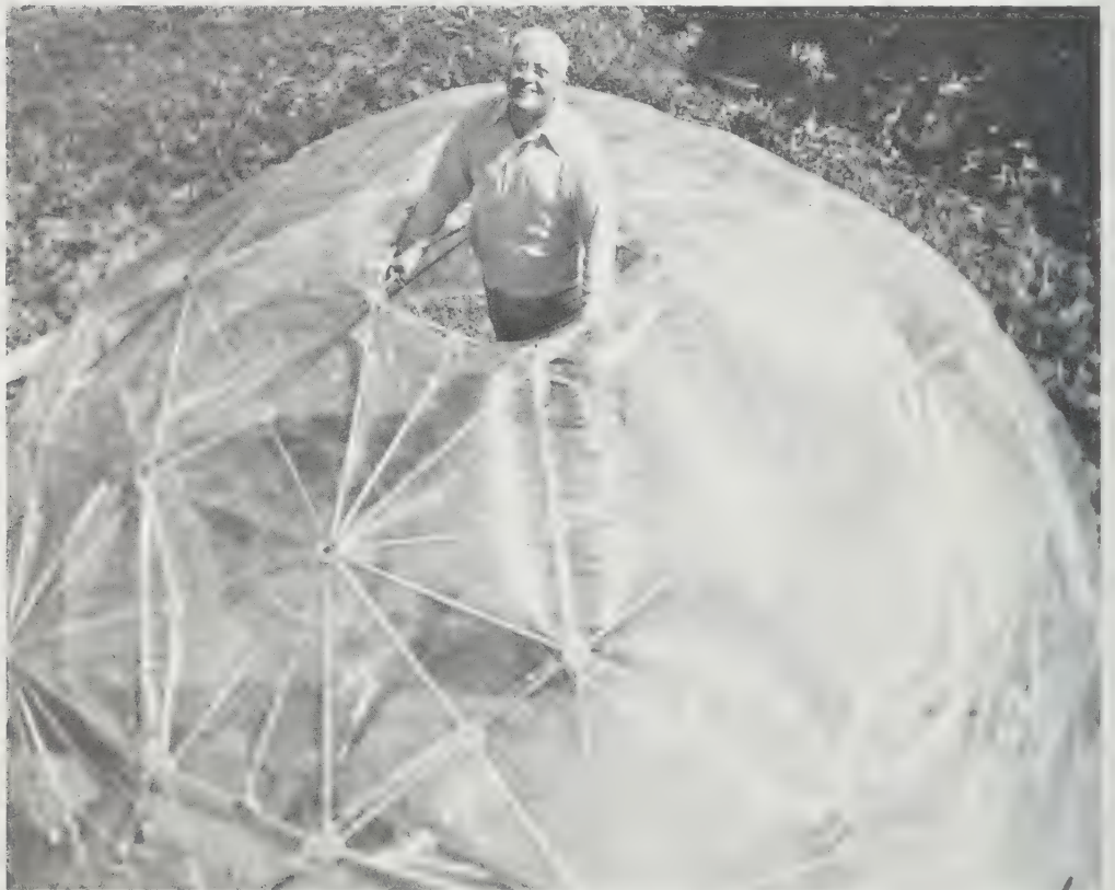
317-318 Same necklace structure erected at Black Mountain College, North Carolina, 1949, demonstrated great strength. When covered with double heat-sealed, pneumatic, transparent skin, the structure maintained, in the sun, an interior temperature 10% below that of the outside air.
