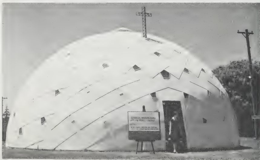
447 Geodesic Plydome chapel of Columbian Fathers adopted by them for leper colonies in the Philippines, Korea, and South Pacific Islands. The chapel has colored plastic windows.
