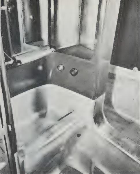
81 View inside bathroom, showing cupboard opened in such a manner that mirror is in use even when door is open. A light was installed along base of mirror. The cabinet provided space for items as large as 5 gallon buckets. Round water control handles were of red and blue plastic. Hot and cold color-coded water handles are now in use on bathroom fixtures in many parts of the world. Note the circular air exhaust grill on lower face of the wall, below the washstand through which steam and stale air were evacuated. The washbasin was without knobs or spigots. The waste handle for the washbasin was a black knob at knee height on the outside of the basin. The drain was actuated by a knob pushed to the right with knee.
