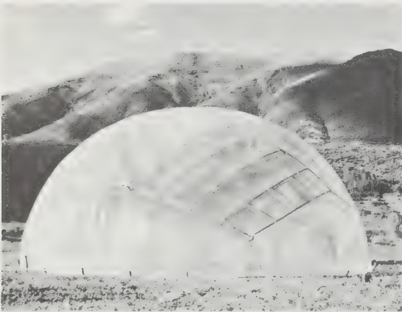
334 Fuller's University of Minnesota students produced 36-foot Geodesic and assembled it in an hour and a half, at Aspen, Colorado, 1952.
