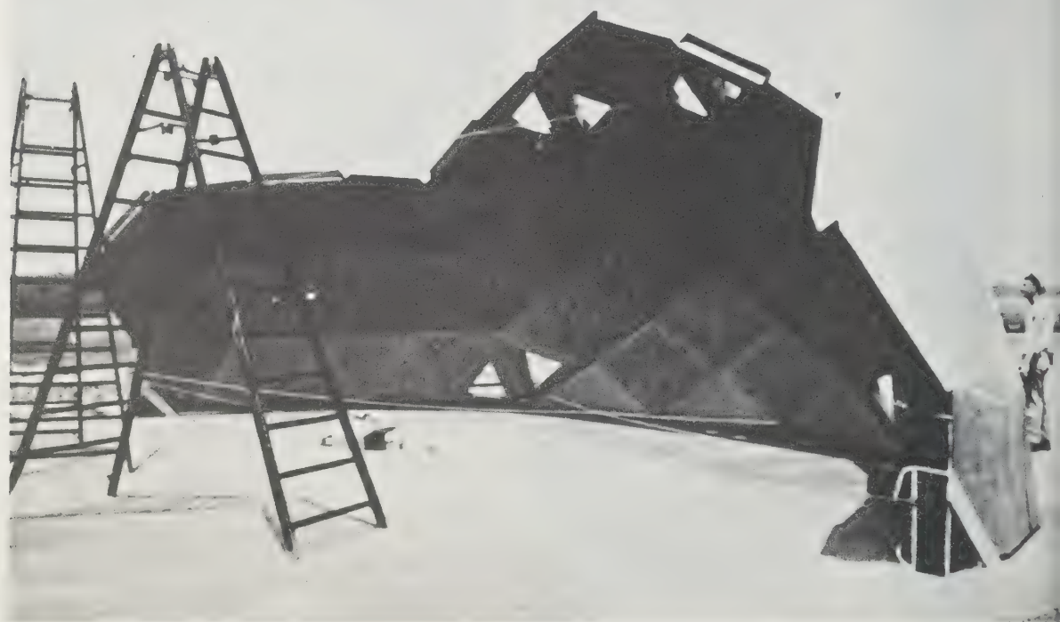
426-430 Printed, scored, and cut blanks for 42-foot, double-skin, paperboard Geodesic dome for U. S. Marine Corps and Triennale of Milan, being assembled at Quantico, Virginia, Marine Corps Base, August, 1954.
