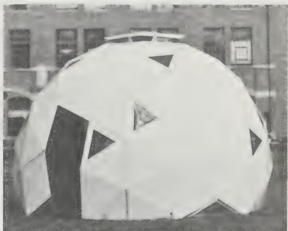
424 Polyester-resin paperboard Geodesic dome, North Carolina State College, 1954.
