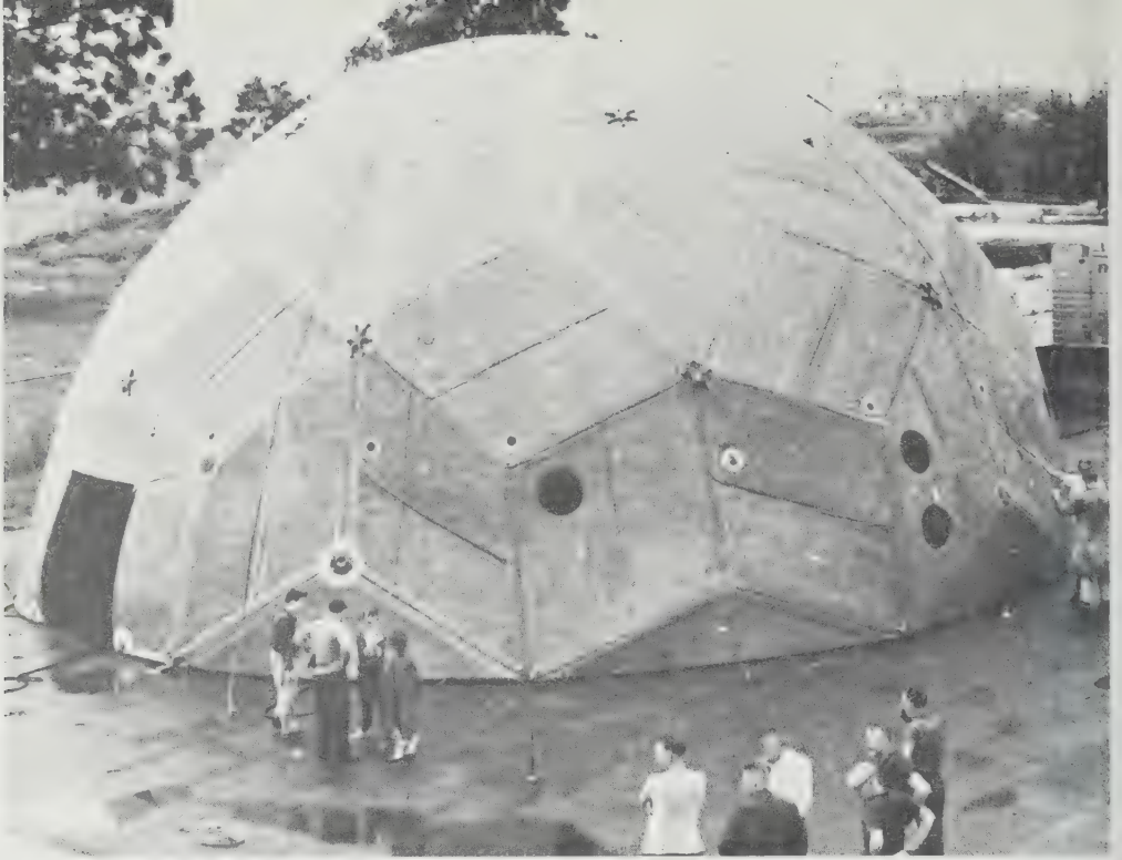
385 Fifty-five-foot, pneumatic, quilted double-skin Geodesic dome, developed and manufactured by Berger Brothers, New Haven, Connecticut, for the U. S. Air Force. A smaller unit by Berger Brothers floated on an ice island to the North Pole as a well insulated personnel shelter.
