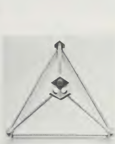
286-287 The Octet Truss can be fashioned from hubs employing the 12 faces of the rhombic dodecahedron. These two pictures show inside and outside of 12-way clevis cluster which holds the ends of struts.
