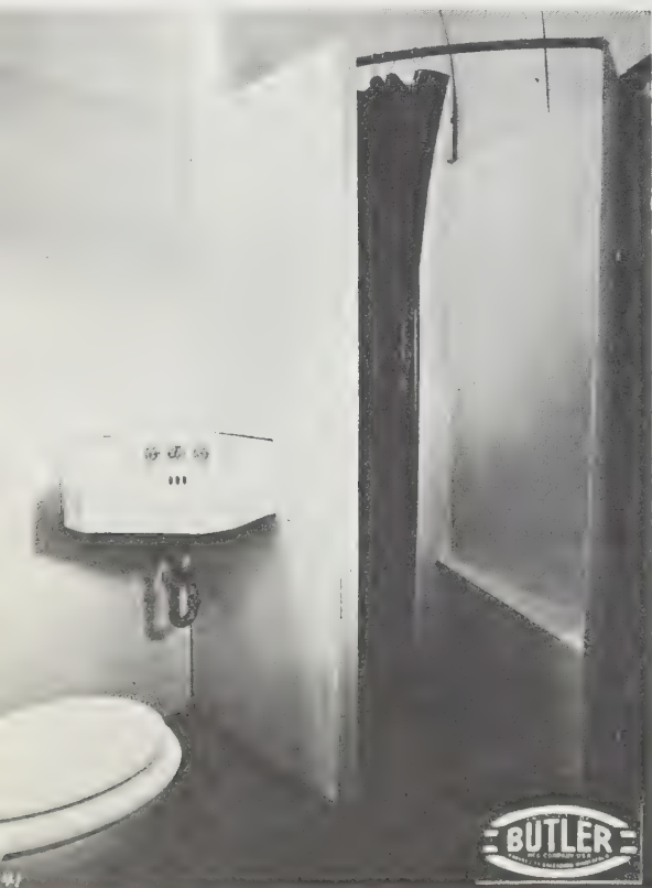
87 Another version of Fuller's Dymaxion Deployment Unit manufactured by the Butler Manufacturing Company, in Kansas City. The seat, basin, and shower, with their flooring and walls, were mounted on a box chassis along with the kitchen plumbing equipment. The latter was placed on the other face of the central wall within which plumbing manifolds, electrical harnesses were installed behind readily demountable panels. (1941)
