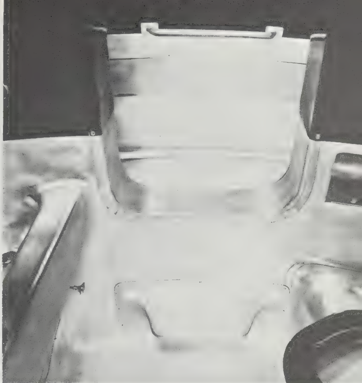
82 Looking into the bathroom from the front door. Note the step for entering the bathtub and shower, at the same level as the bathtub bottom. Handles on either side of door, at entrance to tub and shower area, prevented the possibility of occupant's falling while entering or leaving tub.
