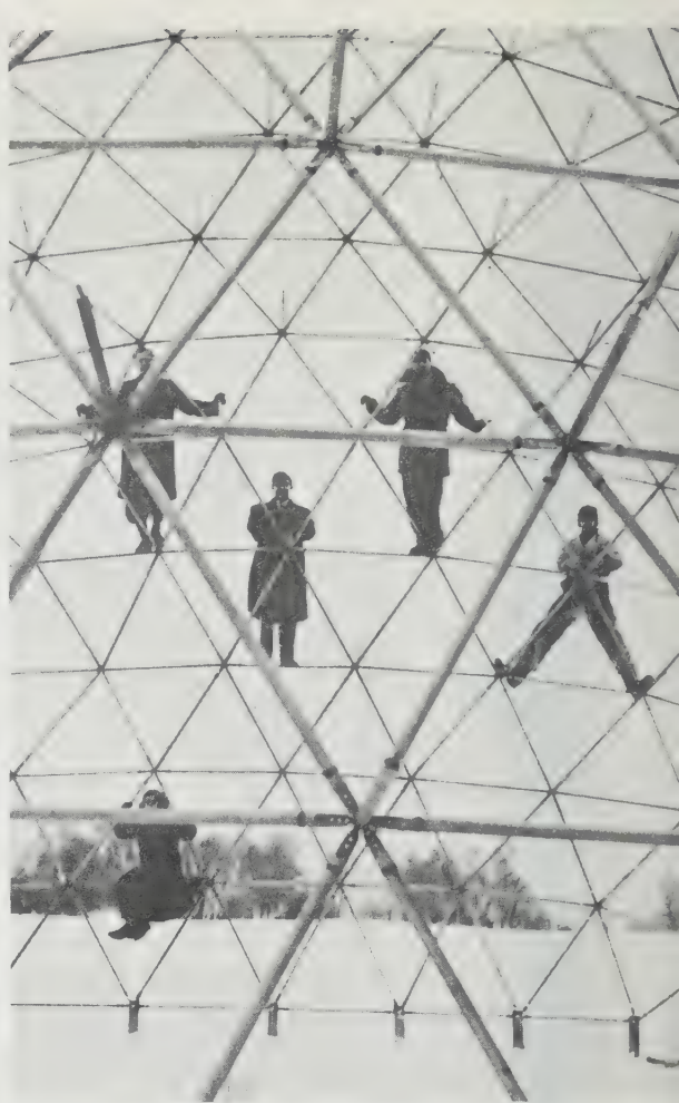
326-328 First large-size (50 feet in diameter) tube and skin structure, erected by the Fuller Research Foundation, Canadian Division, directed and calculated by Fuller's former Institute of Design students, Jeffrey Lindsay and Don Richter, aided by Ted Pope, in Montreal, December, 1950.
