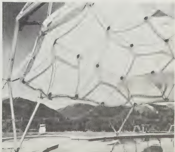
350-351 Magnesium, five-eighths-sphere Geodesic, 42 feet in diameter, erected to cover a naturally-heated swimming pool, Aspen, Colorado, 1954.
