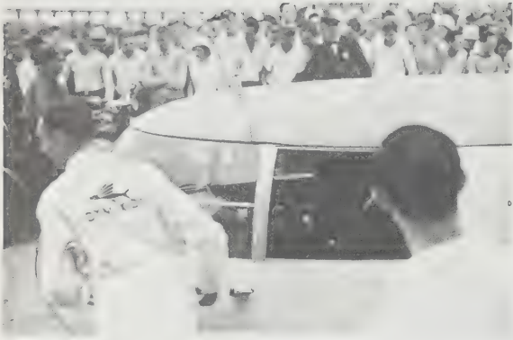
127-128 At Bridgeport, crowds lined the private speedway of the leased Locomobile plant, to watch the first Dymaxion road tests. Extending through the roof above the driver's seat is the car's rear view periscope.
