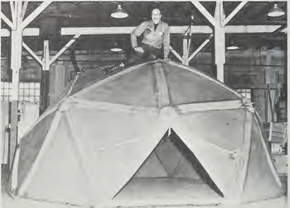
386 A man climbing on the pneumatically firm skin of the Air Force structure. The pressured air is held only within the skin structure, and not inside the dome which opens to the outside through regular doors and windows.
