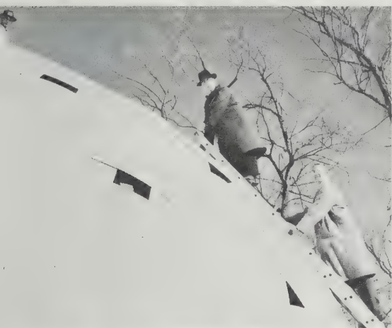
440 Fuller and associates on top of \frac{1}{4} -inch Plywood dome which has no internal frame. Flat sheets that permit five independent axes of bending, together constitute a spherical system when the necessary mathematics have been computed and the indicated join holes punched into boards.
