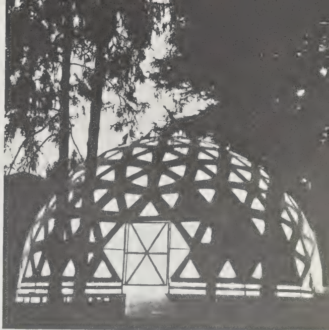
431-433 Forty-two-foot, paperboard Geodesic installed in old Sforza garden, in Milan, where Leonardo da Vinci once worked. The two Geodesic paperboard domes of 1954 (one of which was furnished as a bachelor's apartment) won the Gran Premio of the 1954 Triennale.
