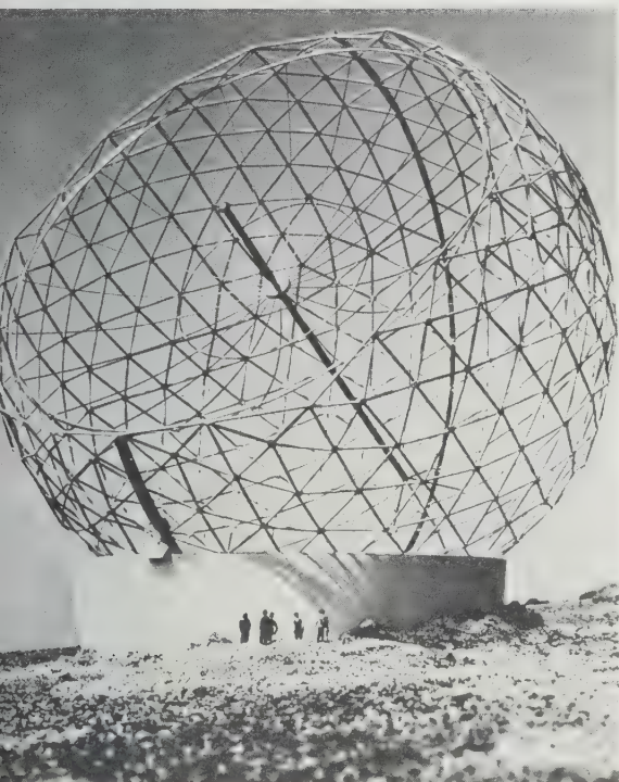
416 Model of parabolic mirrored Sky Eye Geodesic sphere produced in response to U. S. government inquiry preliminary to the development of a radio telescope, 600 feet in diameter.
