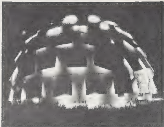
443 "Pine Cone" 42-foot Plydome Geodesic, installed by Fuller and Cornell University students, Ithaca, 1957.
