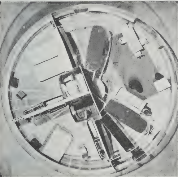
187 View showing the Dwellling Machine's rooms: two bedrooms, two bathrooms, kitchen, entry hall, and living room. The oval pattern of the mechanical enclosures permits a smooth, non-cornered circulation, and a diamond-shaped living room, whose long diagonal was 28 feet.
