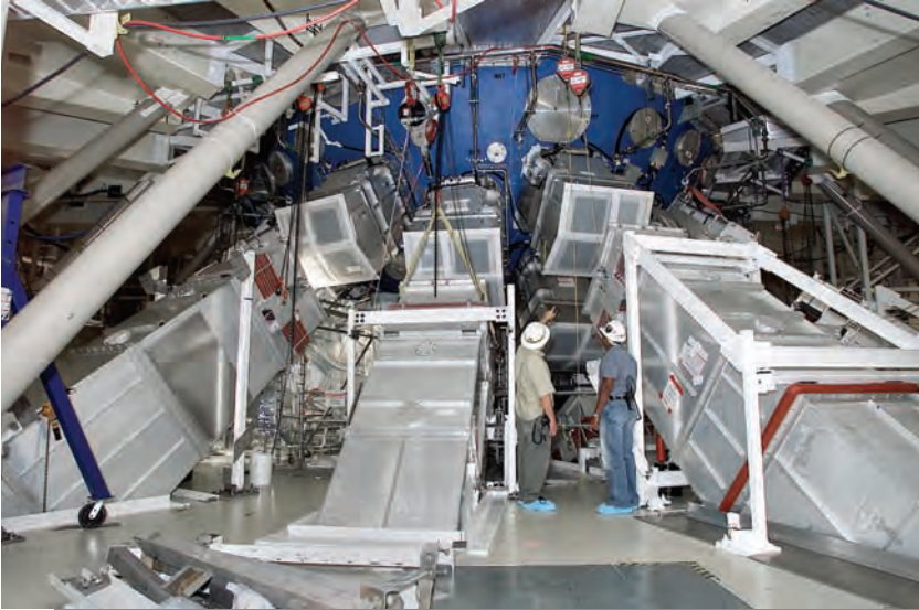
The National Ignition Facility aims 192 laser beams at a small target area. (Lawrence Livermore National Security, LLC, and Lawrence Livermore National Laboratory)
