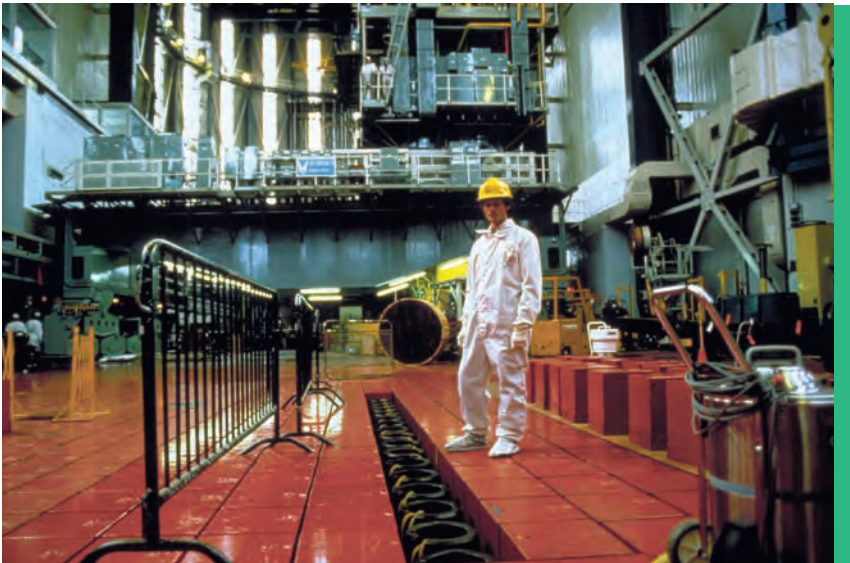
This view of the nuclear reactor at Dungeness B nuclear power station in Kent, England, shows the top of the plate in which uranium fuel rods are housed. (Jerry Mason/Photo Researchers, Inc.)
