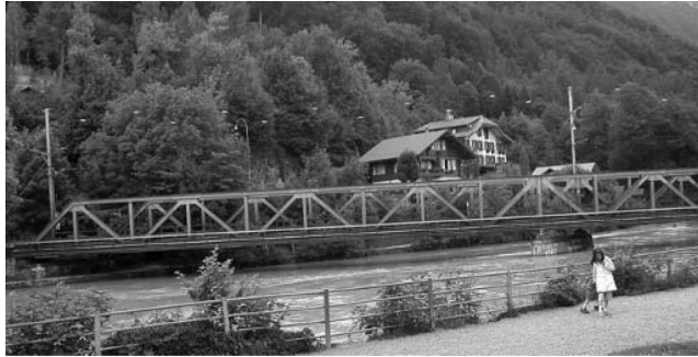
FIGURE 12.10 Truss Bridge in Interlaken, Switzerland
