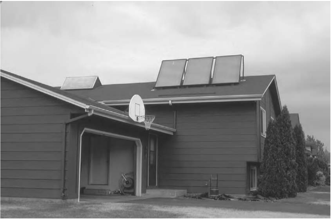
Solar panels on a home (Michael Siluk)
