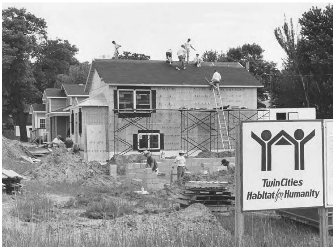
Habitat for Humanity volunteers building homes (Michael Siluk)
